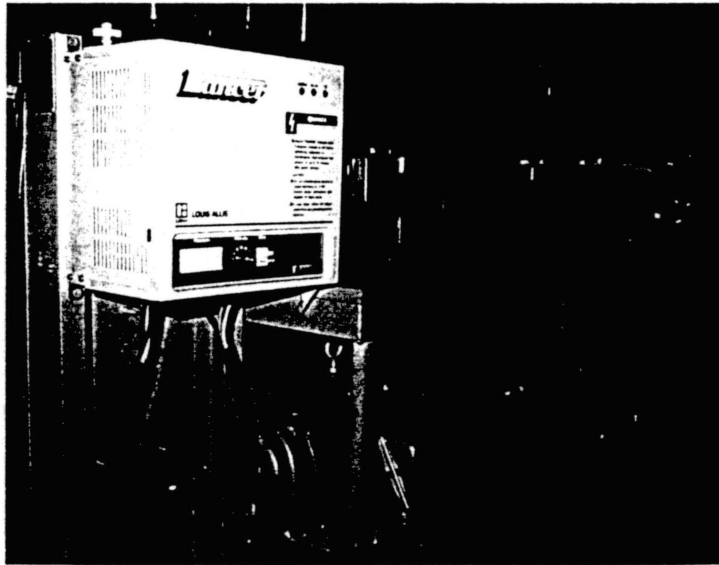
Figure 16. Variable Speed Drive Controller
