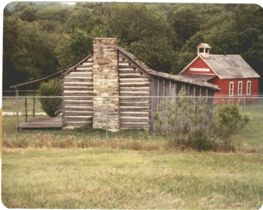
Figure 12. East Elevation, Kerr Cabin
