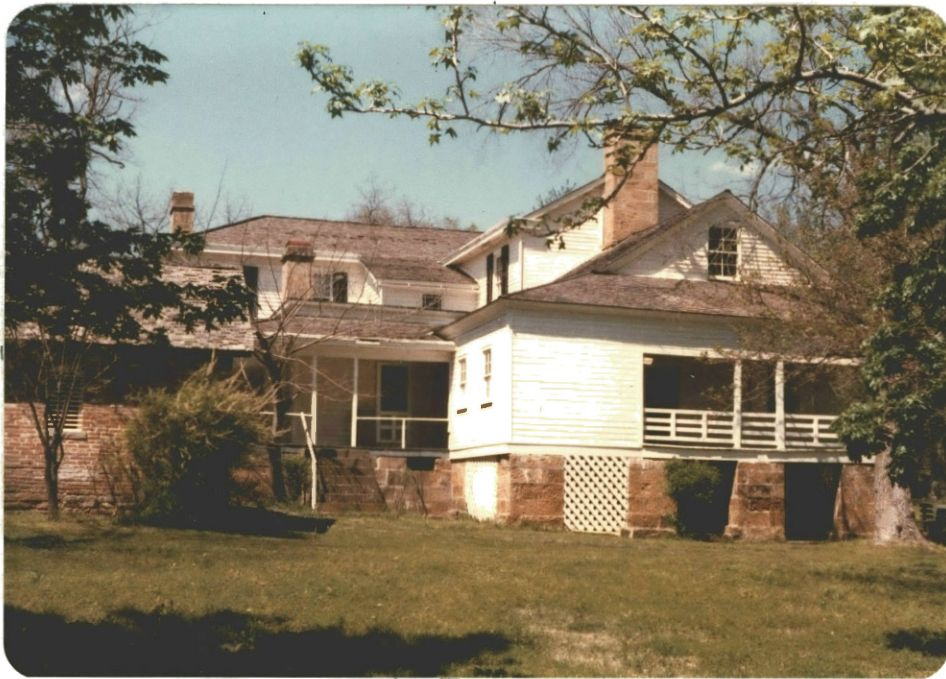
Figure 4. South Elevation, Hunter's Home
