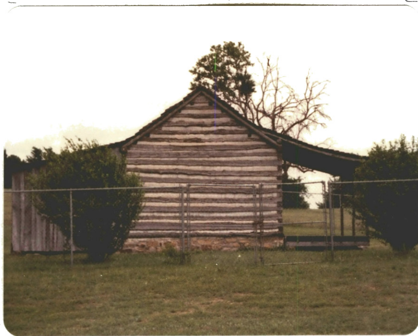
Figure 14. West Elevation, Kerr Cabin
