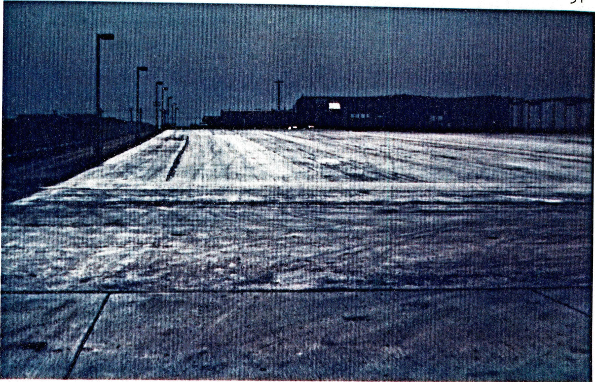
(a) Immediate Foreground, PCC; Remainder Completed RCC
