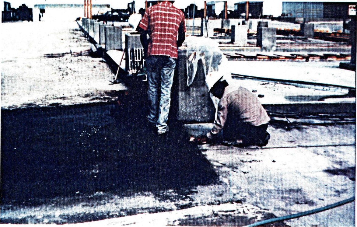
(a) Using Hand Compactor in Tight Areas
