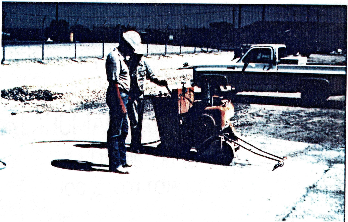
(b) Concrete Saw Used for Joints and Waste Removal
