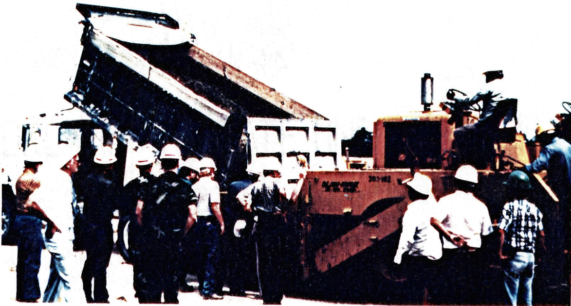
(b) Dumping of First Load of RCC
