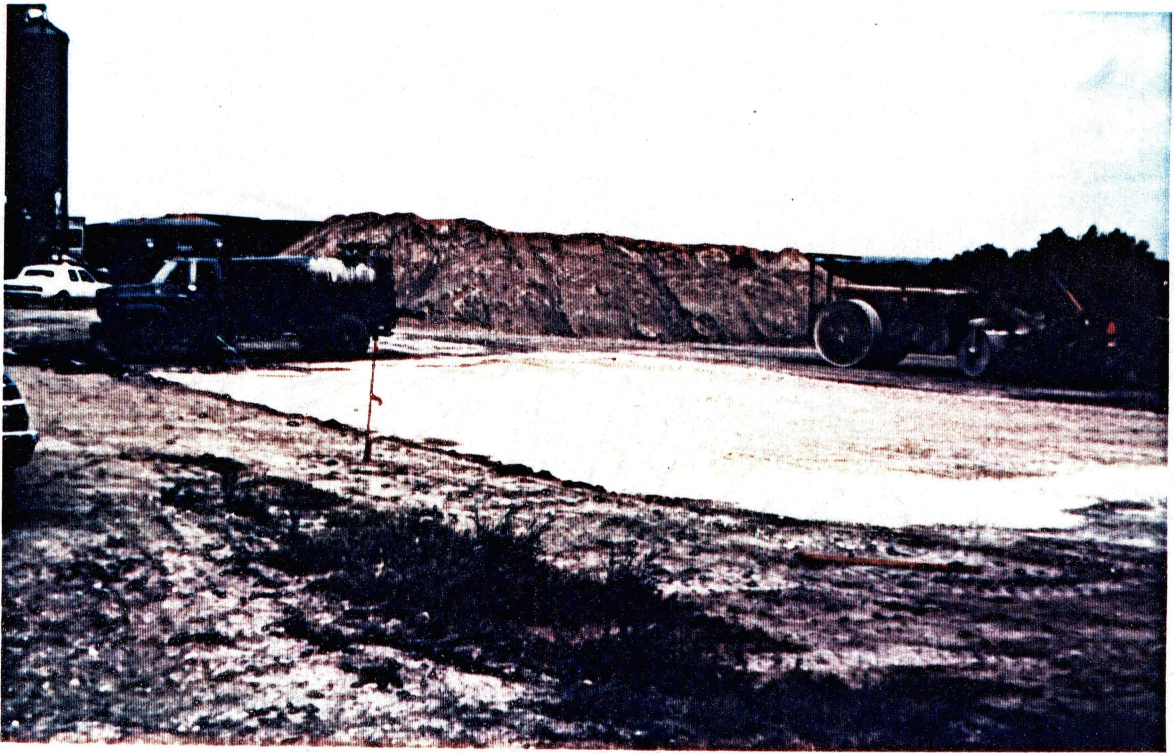
(a) Prepared Foundation for Test Section
