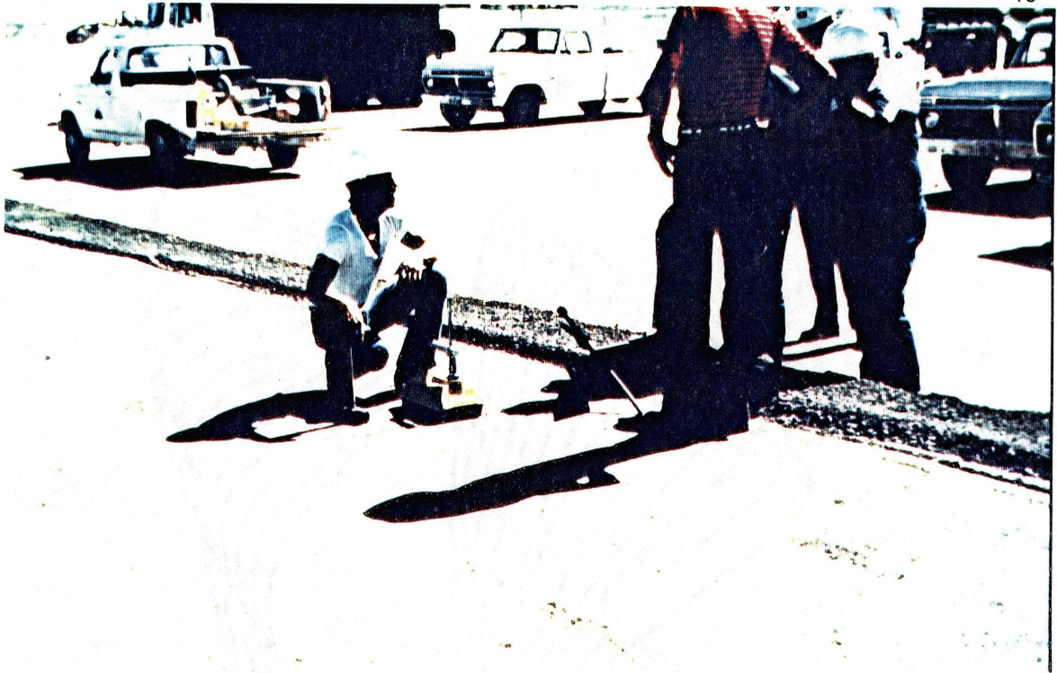
(a) Using Troxler Road Reader
