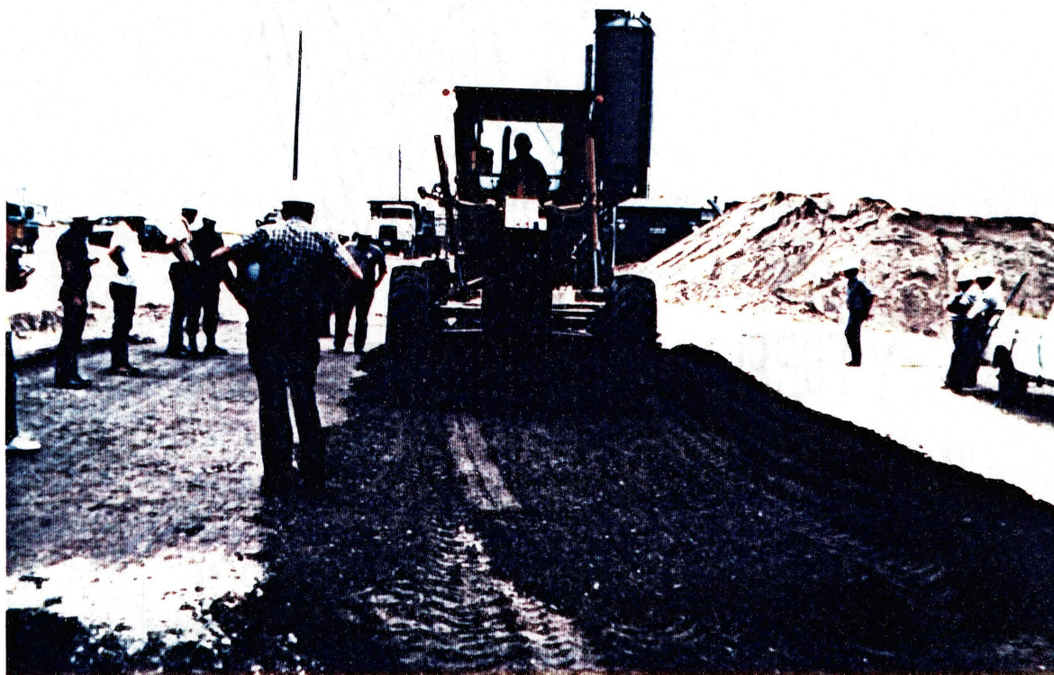
(b) Second Lane, Two-Lift Construction
