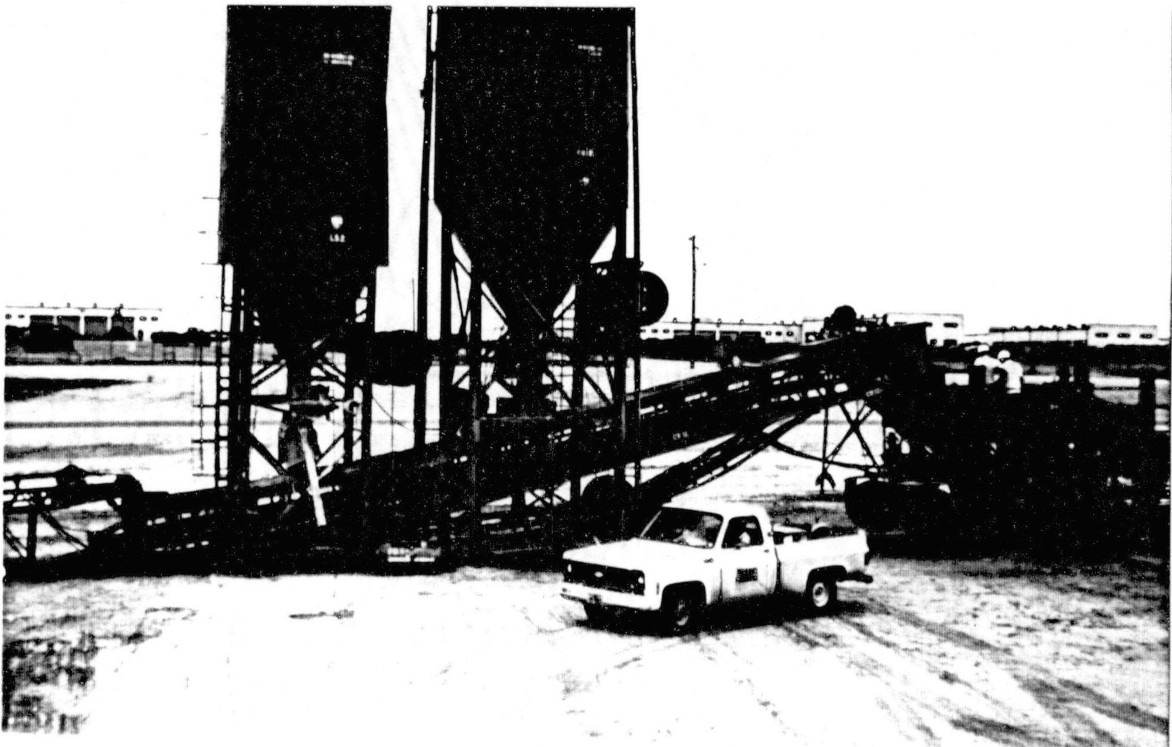
(b) Silos and Pugmill
