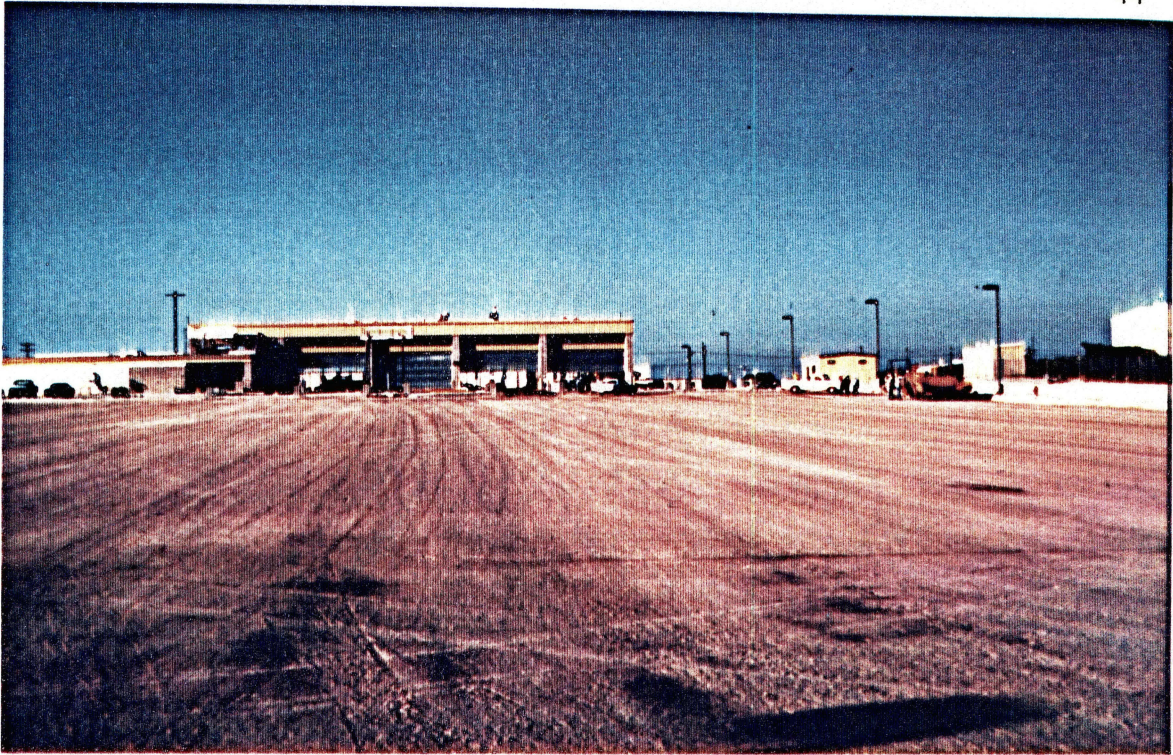
(a) Prepared Foundation Before Placement Began
