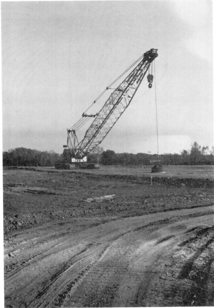
Figure 18. Photograph of Crane Used on Project
