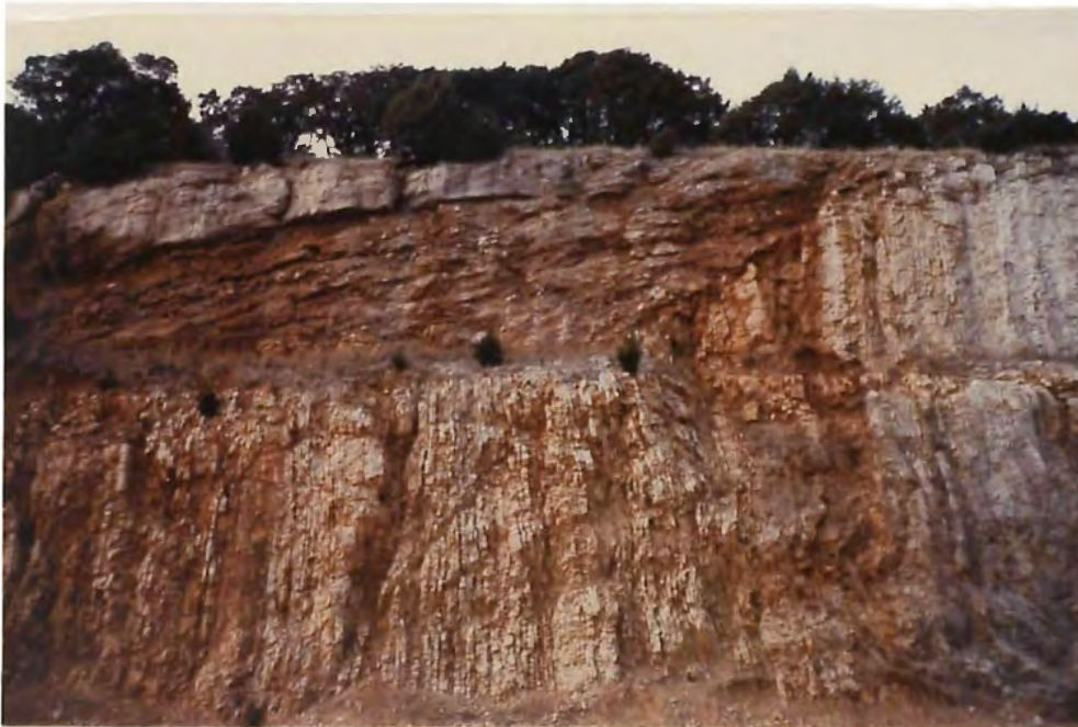
Figure 7. Angular unconformity between the Pennsylvanian Collings Ranch Conglomerate (top of photograph) and vertical Ordovician Viola Limestone (bottom of photograph), I-35 roadcut.
