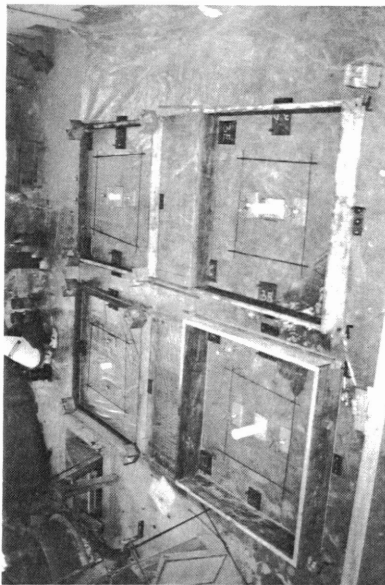
Figure 10 Position of PVC Pipe and Concrete Inserts
