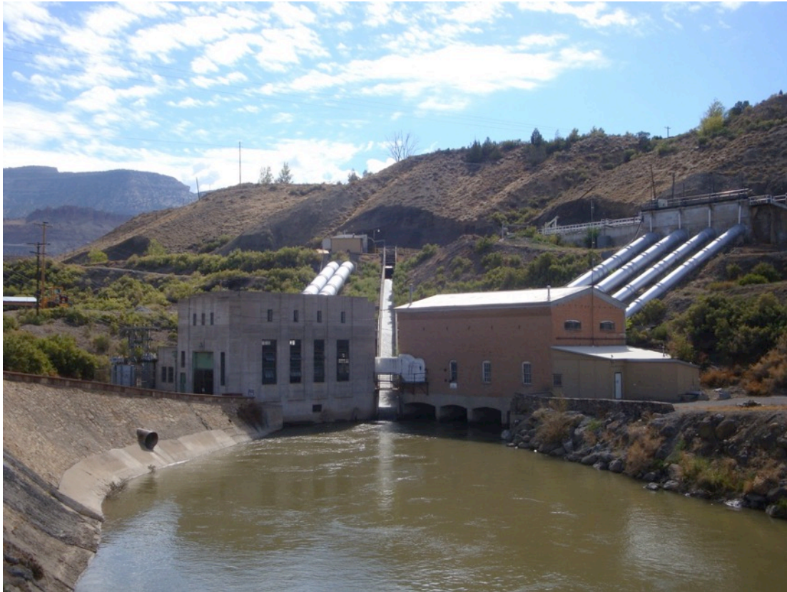
Figure 26. OMID pump house (on the right) and power plant (on the left).
