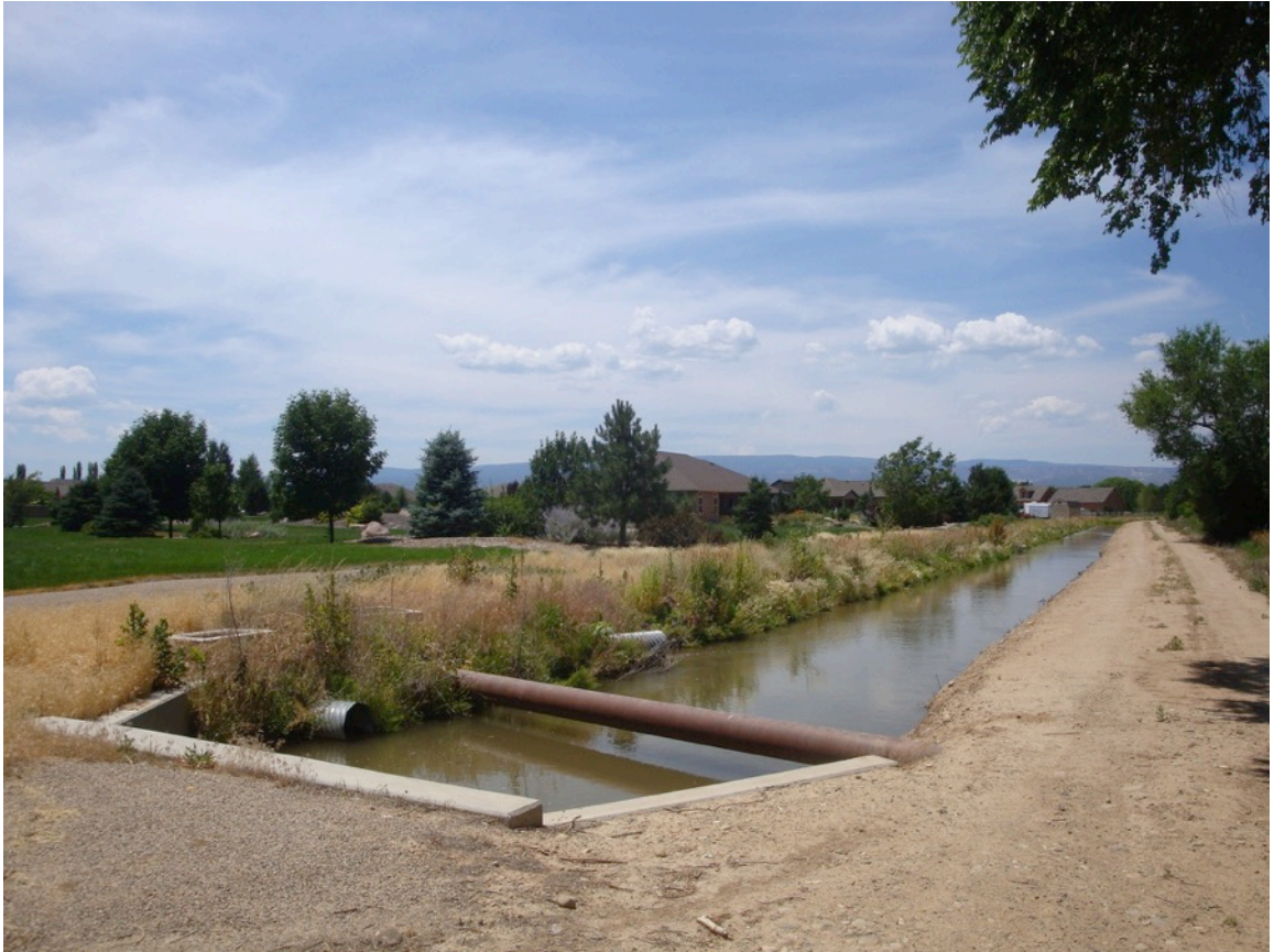
Figure 32. Large homes are going up south of Rettig Farms.
