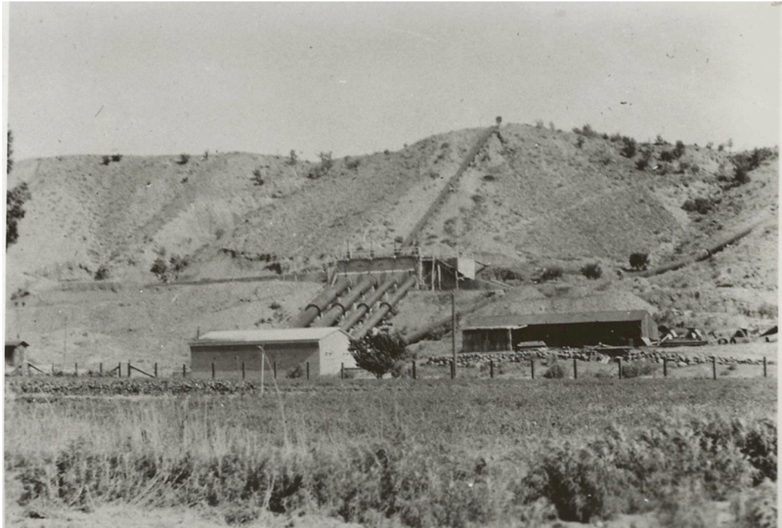
Figure 25. OMID pump house, circa 1900. 15
