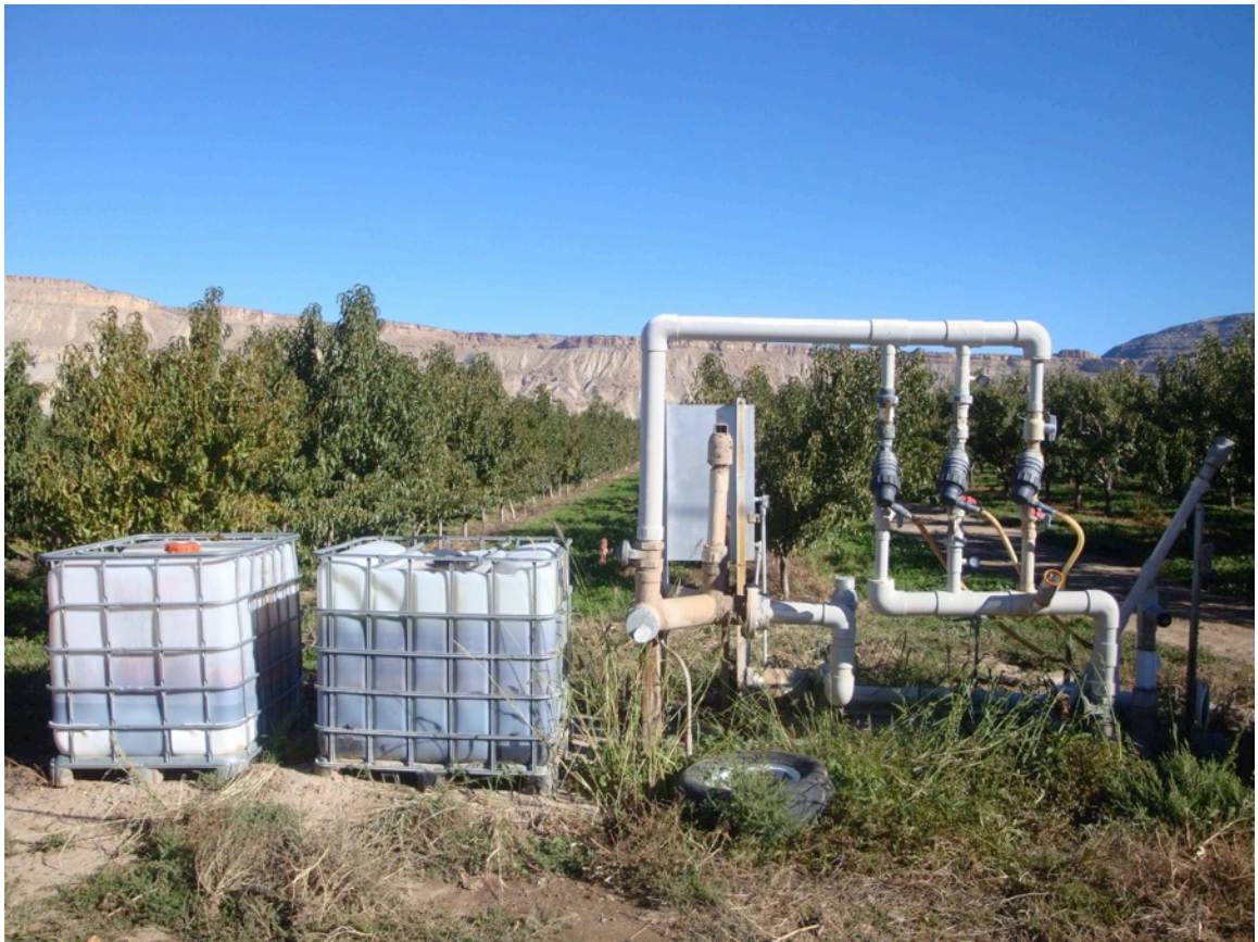
Figure 28. C&R #2 micro-jet irrigation system.
