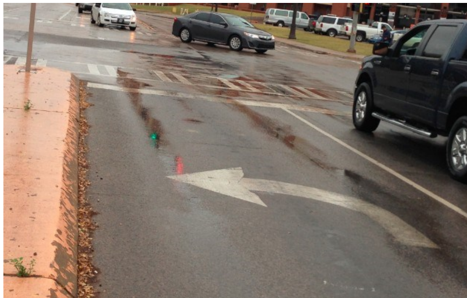
b. An Example of Rut at Intersection with Pooled Water
