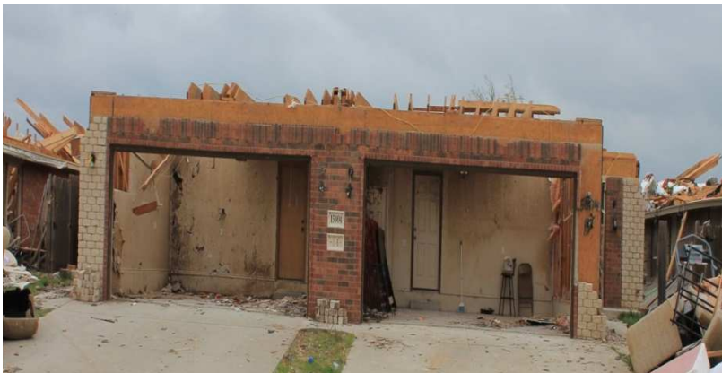
Figure 2: Roof Failure
