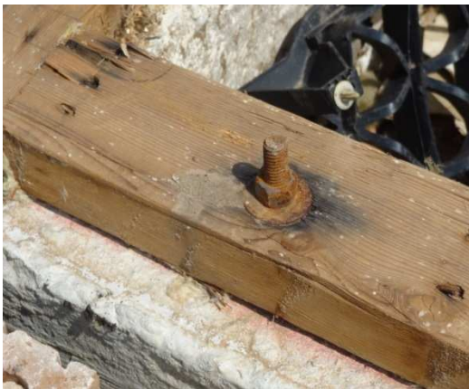
Figure 4: Bottom Plate Anchored to Foundation
