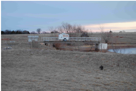
(a) View of bridge deck looking to the South-east
