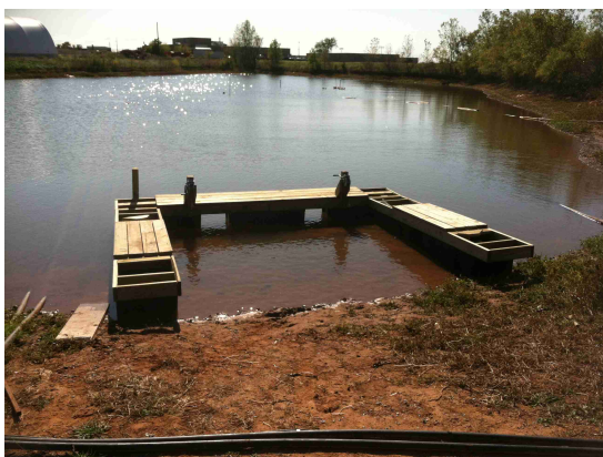
(c) Third segment of ice-on-coil platform.
