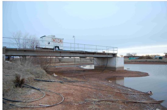
(b) Close view of bridge deck
