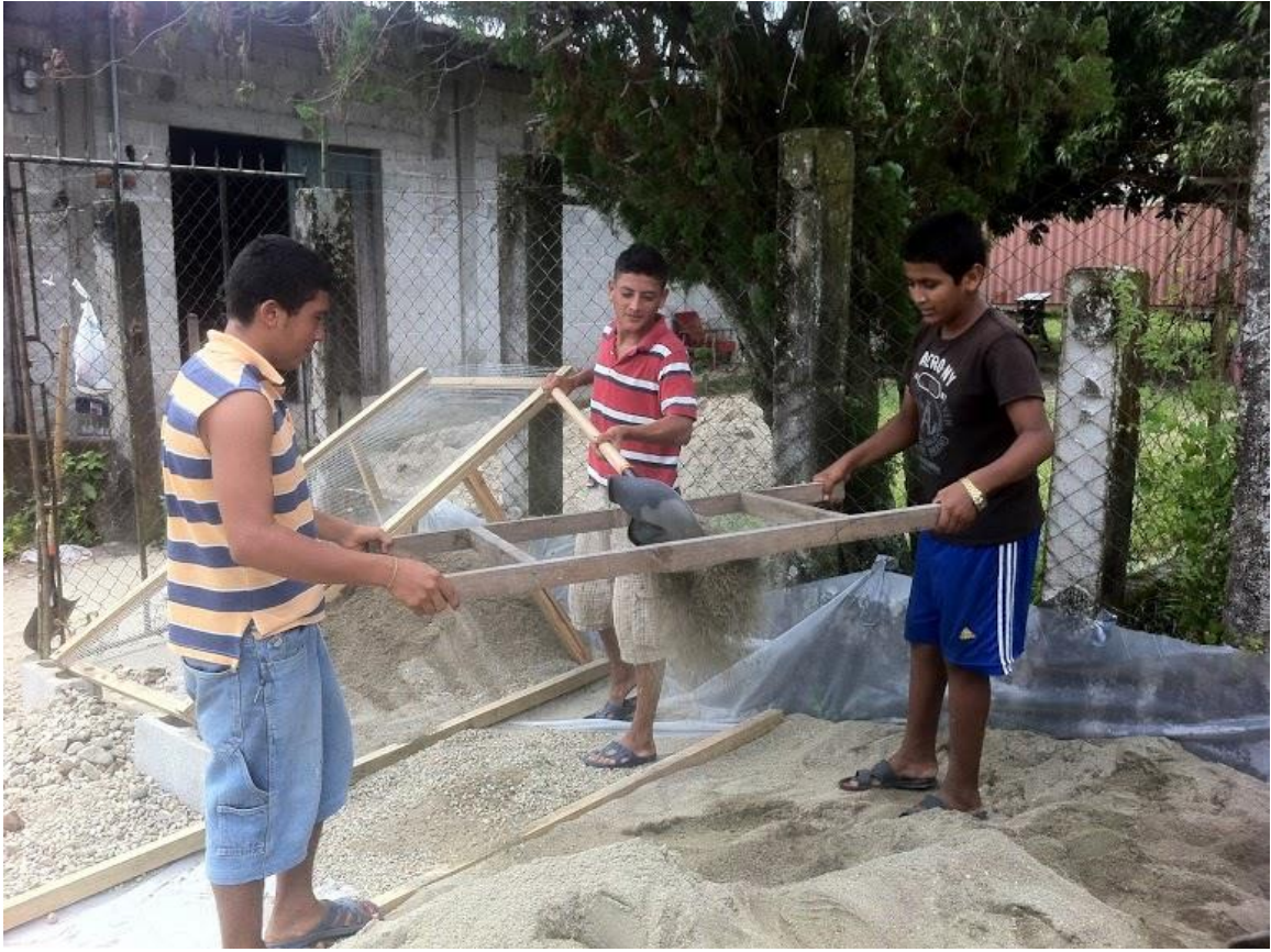
Figure 21: Swinging Sieving Method
