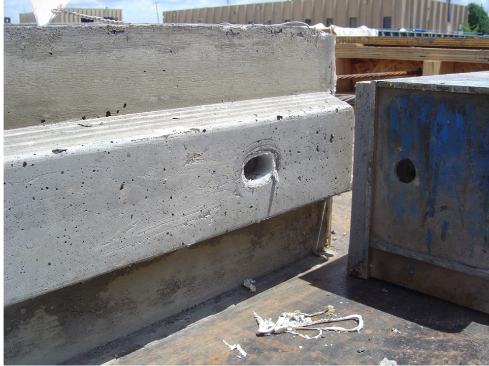
Figure 20 Shear key and the two-strand post-tensioning duct
