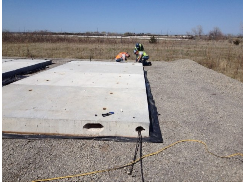
Figure 34 Strand threaded manually through ducts for Pavement III
