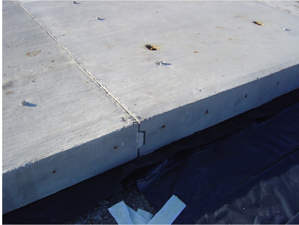
Figure 31 Panels shear key at joint
