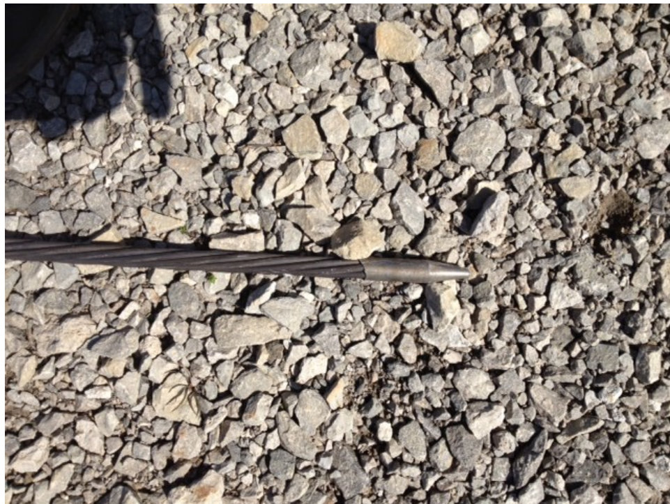
Figure 35 Hardware used at strands tip for better threading
