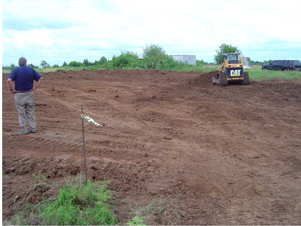
Figure 23 Project site subgrade preparation
