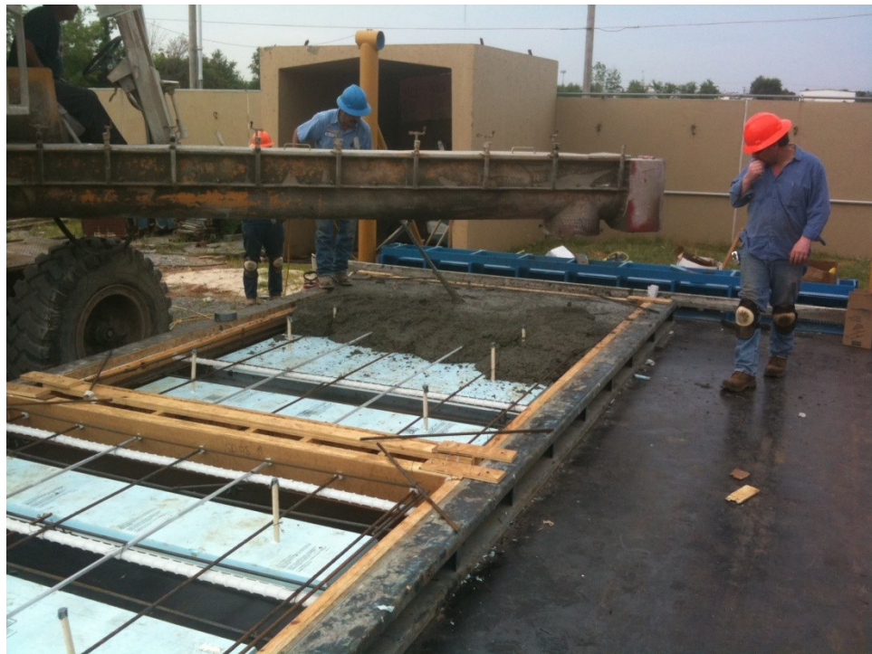
Figure 17 Concrete cast into panel form
