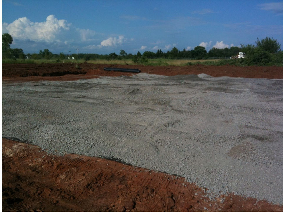
Figure 26 Base materials preparation and leveling
