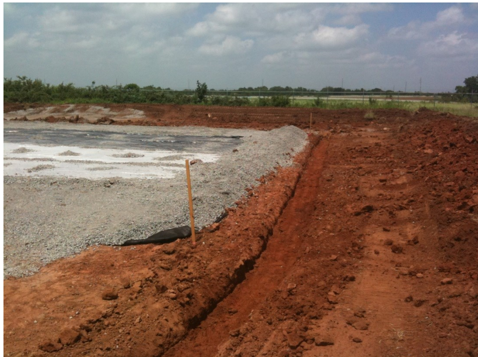
Figure 28 Storm water drainage all around test area
