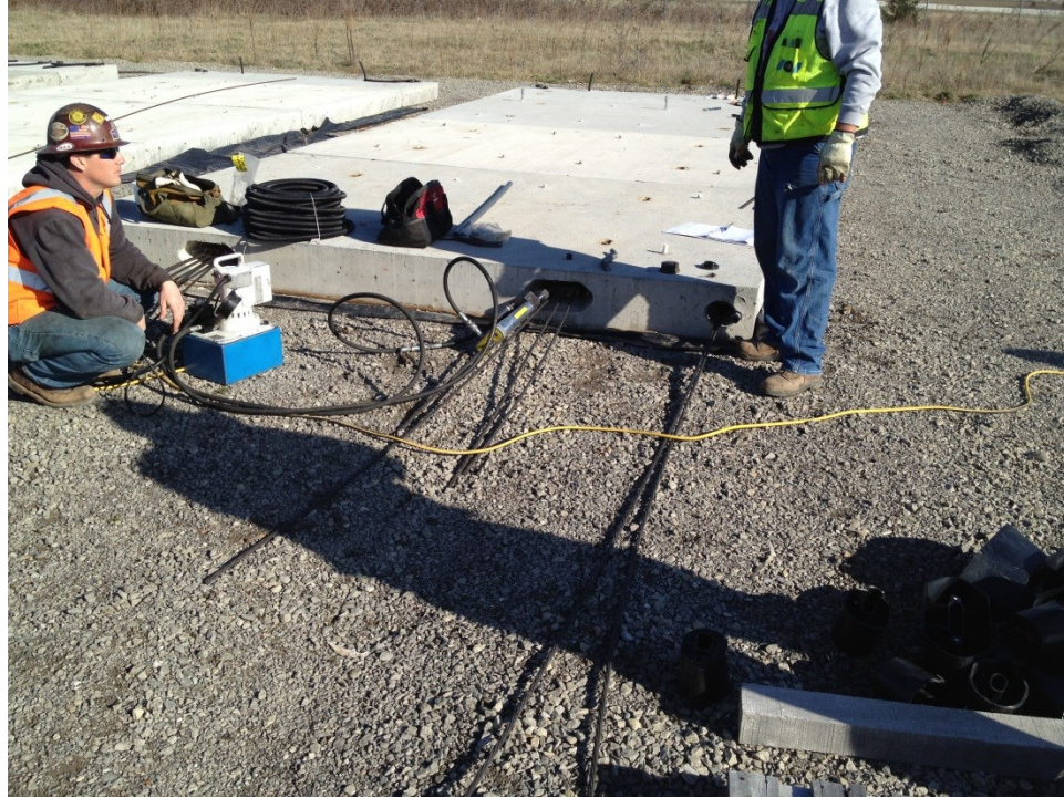
Figure 36 Tendons stressing for Pavement III
