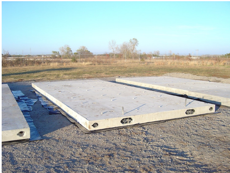
Figure 32 Pavement panels assembled and ready for post-tensioning
