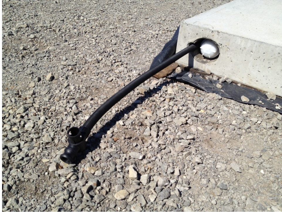
Figure 38 Sealed anchor with grouting hose for two strand system
