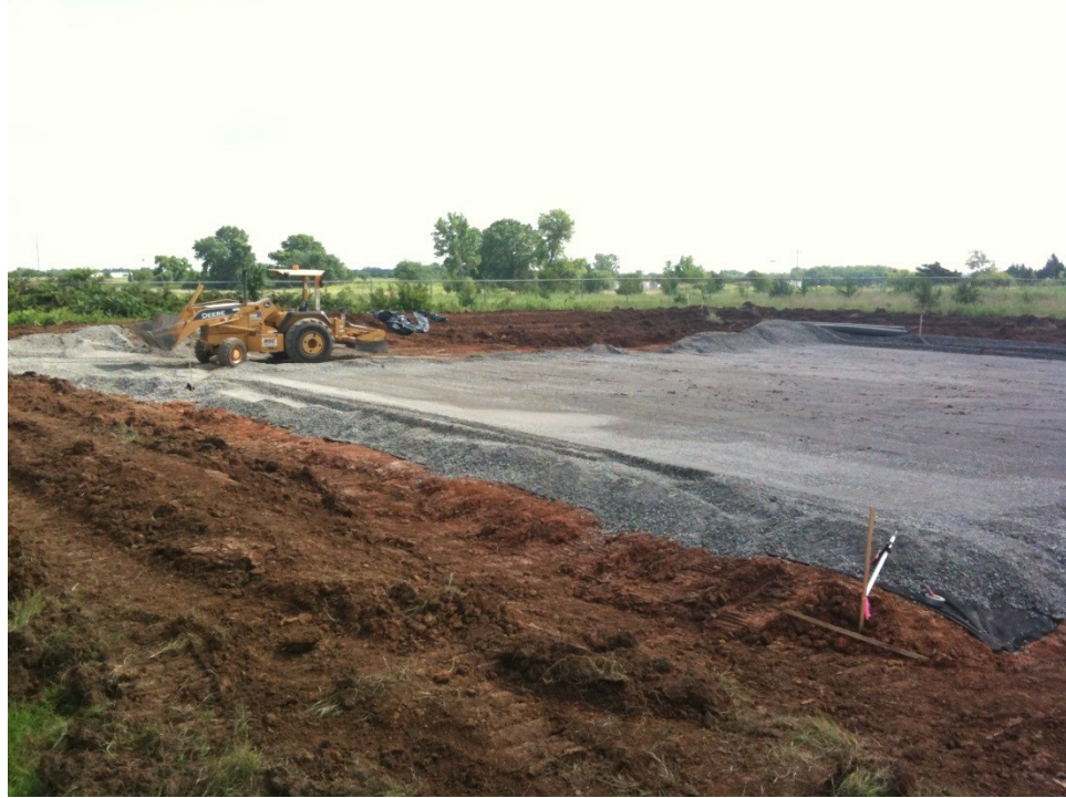
Figure 27 Base grading and compaction
