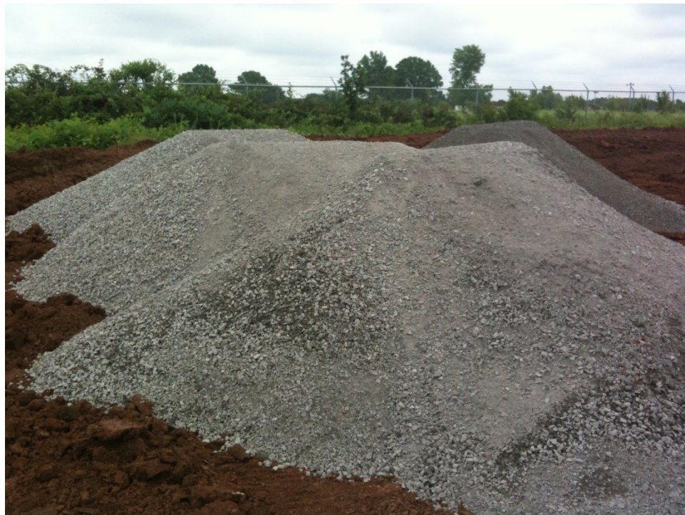
Figure 24 Aggregate base material delivered to site
