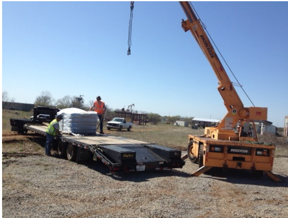
Figure 33 Grout being delivered to jobsite
