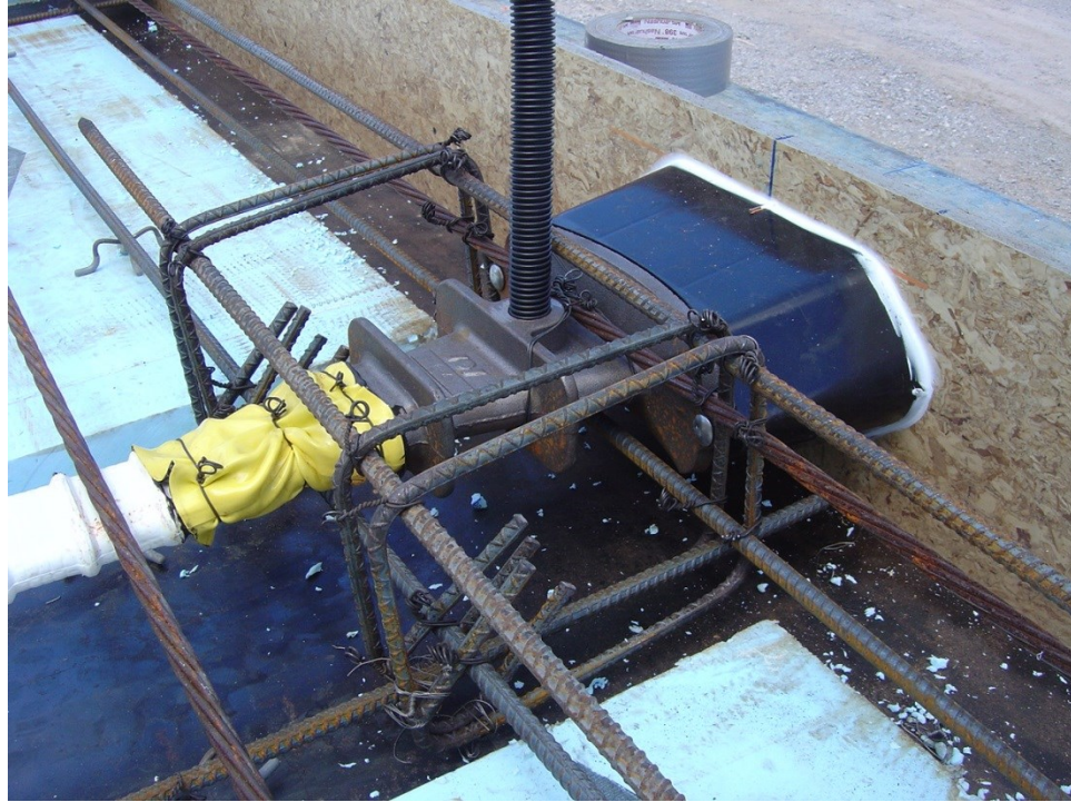
Figure 16 Post-tensioning hardware for 4-strand anchors
