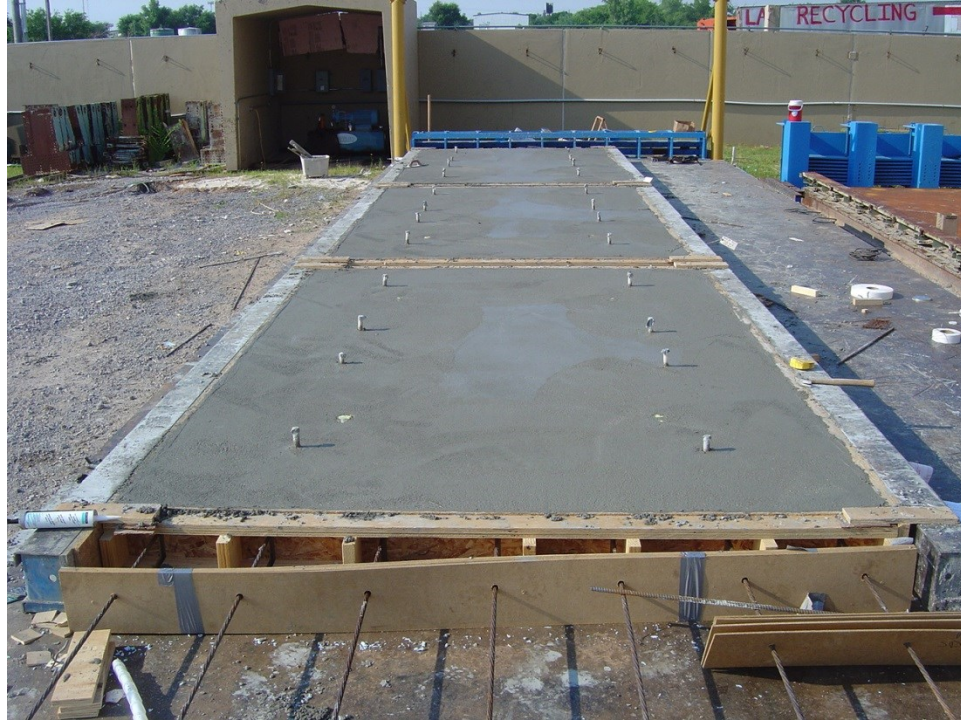
Figure 18 Finished panel surface
