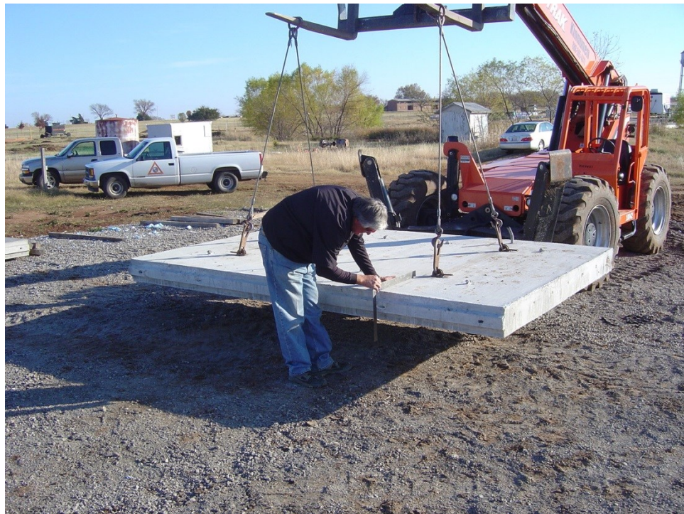
Figure 30 Marking ducts location for alignment
