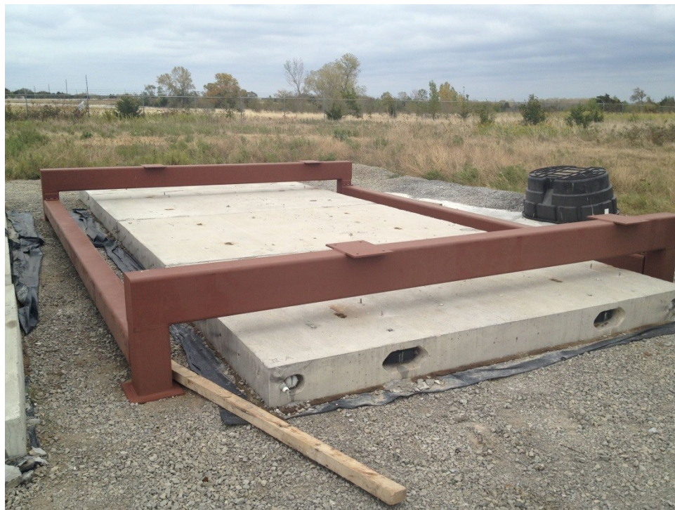
Figure 44 Base frame assembled on site over Pavement III
