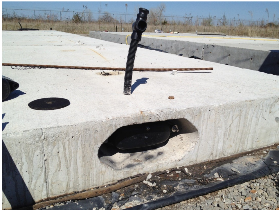
Figure 39 Sealed four strand anchor head with grouting house for Pavement II
