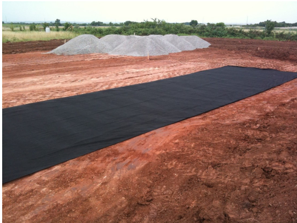
Figure 25 Road fabric prior to placing aggregate base
