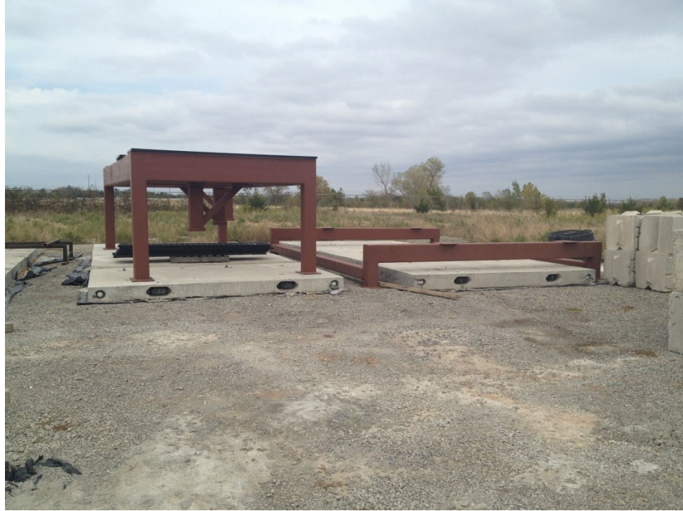
Figure 45 Top and base frame prior to assembly
