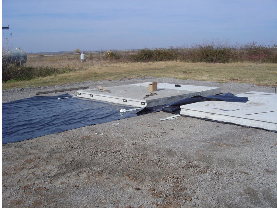
Figure 29 Panels placement on friction reducing membrane
