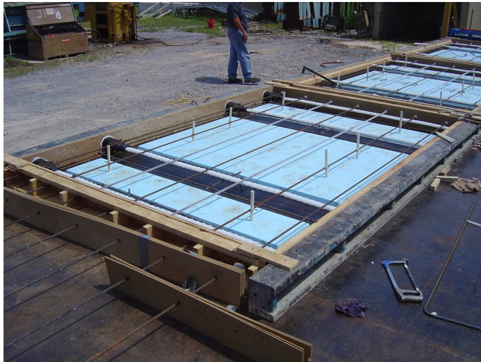
Figure 15 Concrete formwork for Panel I-A
