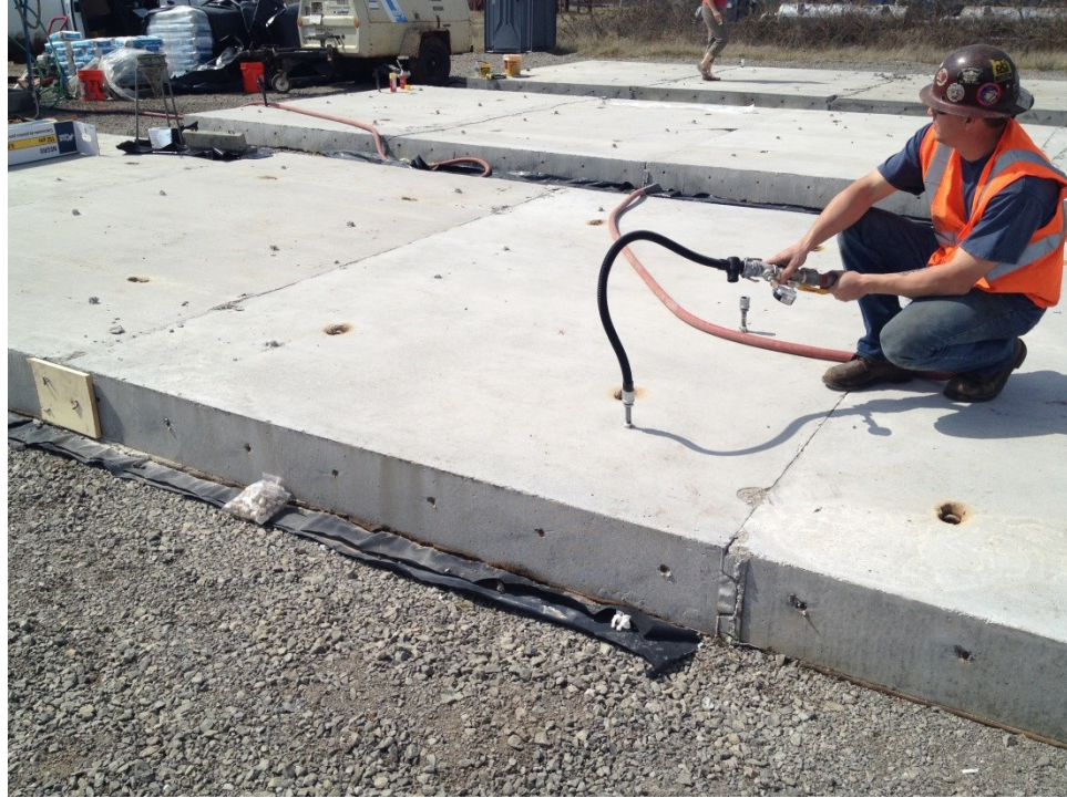
Figure 40 Grouting under panel pockets for Pavement III
