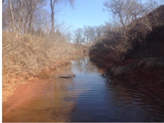
Figure F.11.4: FGM Site NF-02 – Bank 1 - Looking downstream (rt).
