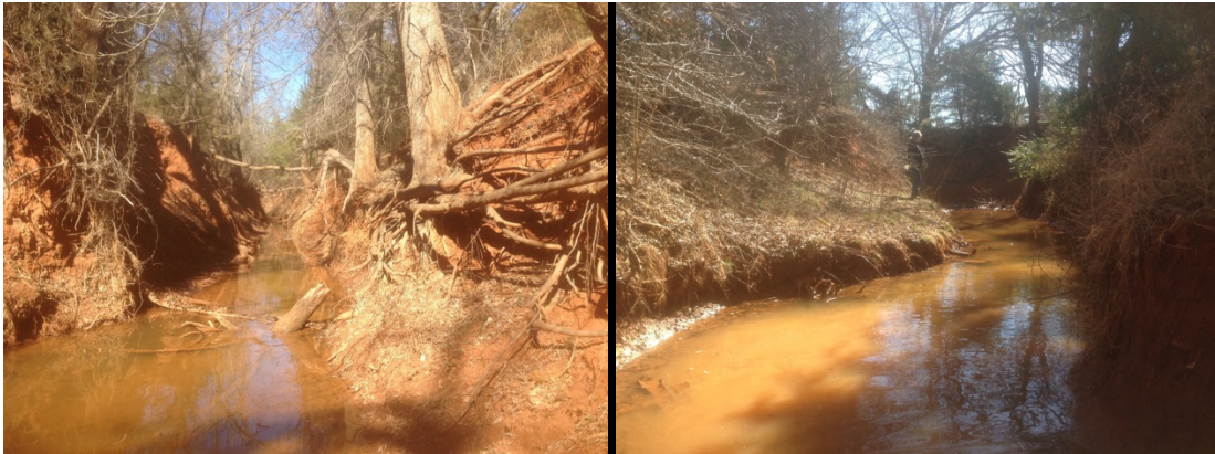
Figure F.19.1: FGM Site RC-04 – Cross Section - Looking upstream (lt); Looking downstream (rt).
