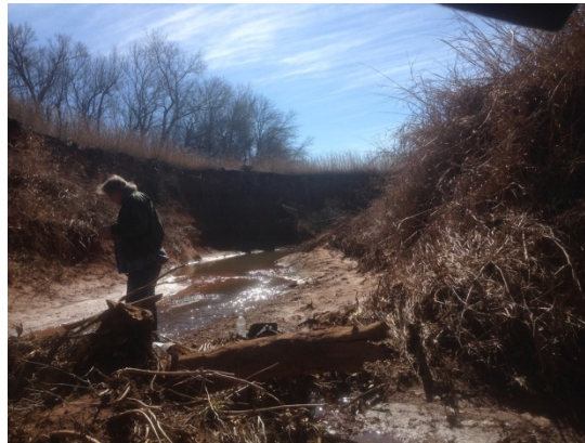
Figure F.7.8: FGM Site LR-07-Bank 4–Facing upstream.
