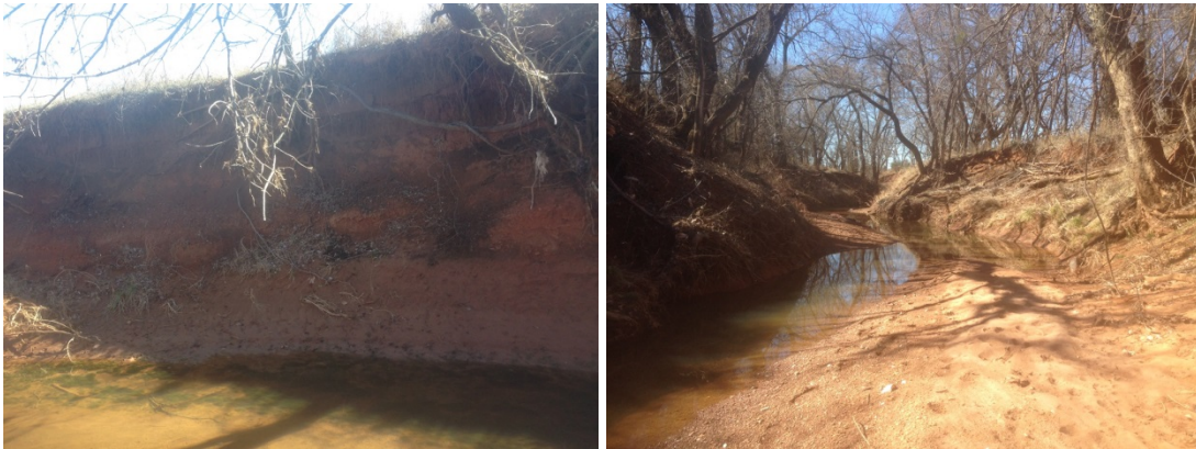
Figure F.9.6: FGM Site LR-09 – Bank 3 - Bank (lt); Facing upstream (rt).
