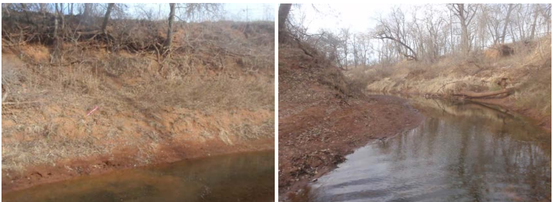
Figure F.2.6: FGM Site LR-02 – Bank 3 - Bank (lt); Facing upstream (rt).
