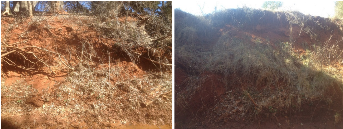
Figure F.19.2: FGM Site RC-04 – Cross Section - Left Bank (lt) – Right bank (rt).
