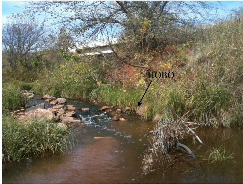
Figure A.5.2: Elm Creek at Indian Hills (SE 179 th ) monitoring site HOBO installation.
