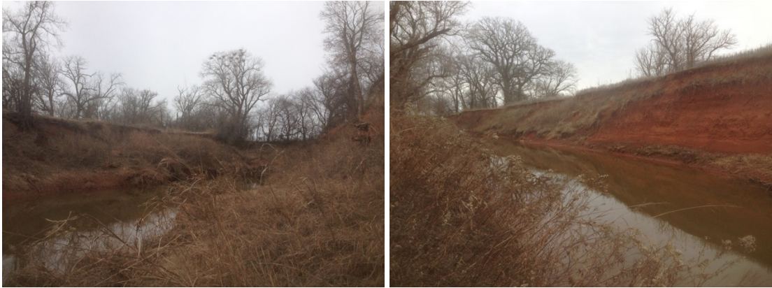
Figure F.4.5: FGM Site LR-04–Bank 2-Facing upstream (lt);Facing downstream (rt).
