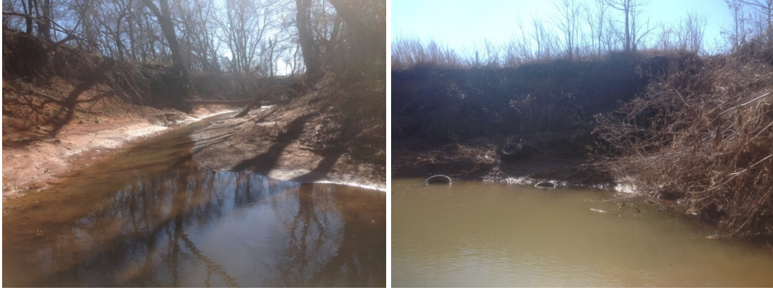
Figure F.7.4: FGM Site LR-07 – Bank 1-Facing downstream (lt); Bank 2-Bank (rt).
