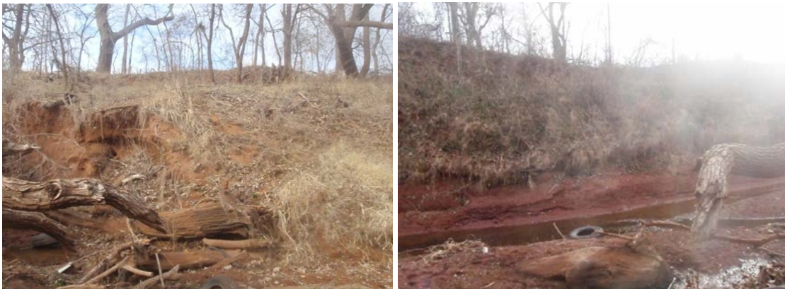
Figure F.2.2: FGM Site LR-02 – Cross Section - Left Bank (lt) – Right bank (rt).
