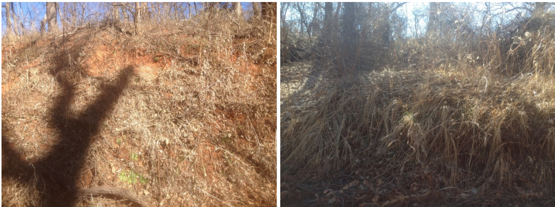
Figure F.17.2: FGM Site RC-01 – Cross Section - Left Bank (lt) – Right bank (rt).
