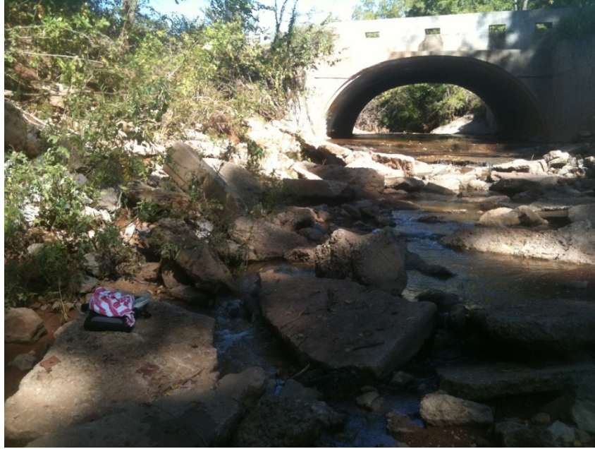
Figure A.6.2: North Fork at Franklin monitoring site HOB0 installation.
