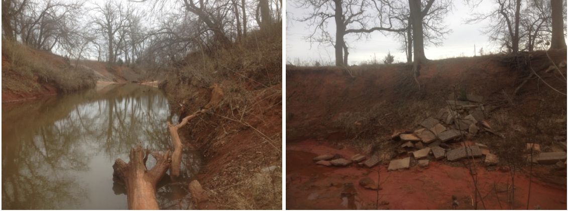
Figure F.4.7: FGM Site LR-04 – Bank 3–Facing downstream (lt); Bank 4-Bank (rt).
