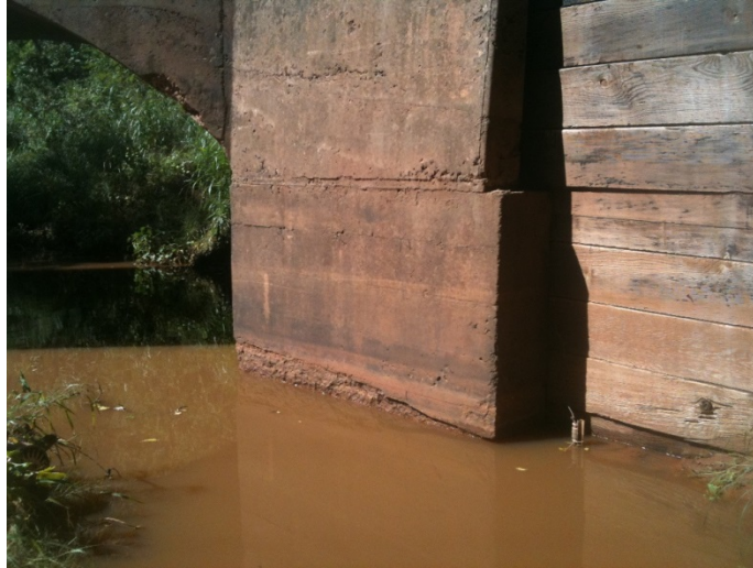
Figure A.4.2: Rock Creek at 72 nd Ave NE site HOBO installation.
