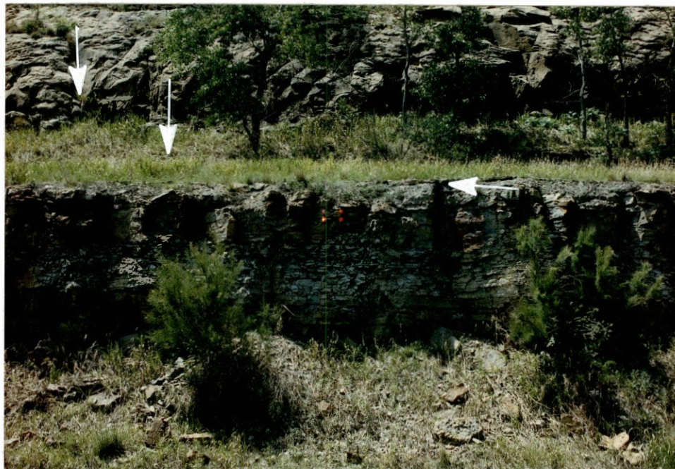
Figure 14: Photograph of the outcrop location of a throughgoing fault in the Lecompton Limestone near Oilton. Arrows indicate the position of the fault and the location of the close-up photograph in Figure 15.
