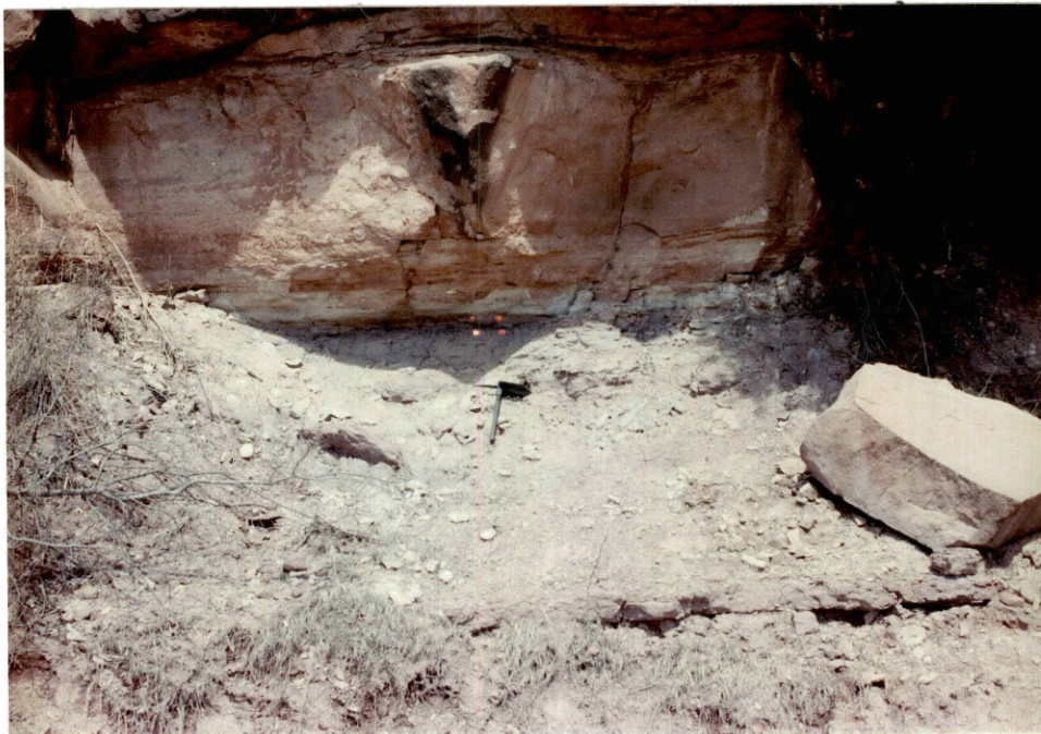
Figure 16: Photograph of a portion of the outcrop at Ripley showing a jointed sandstone overlying shale. (Camp shovel is approximately 24 inches long)
