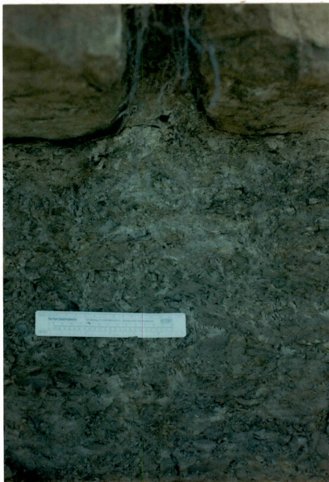
Figure 23: A close-up view of the main joint seen just left of the Jacob staff in Figure 22. The joint ends abruptly at contact with shale. (Ruler is 6 inches long.)
