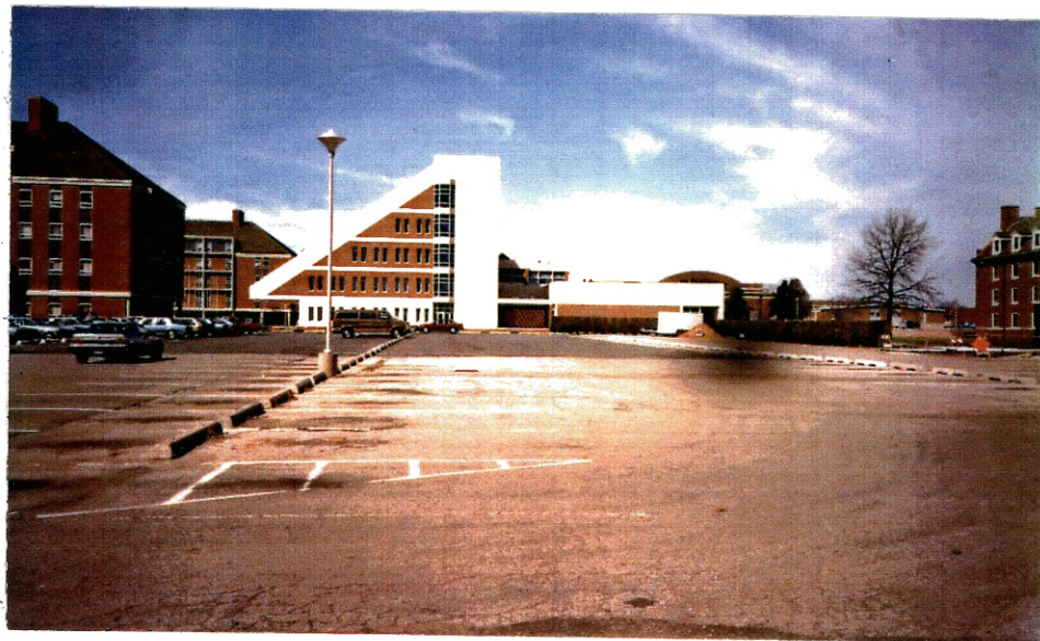
Figure 39. Newly Refurbished Temporary Lot 11.
