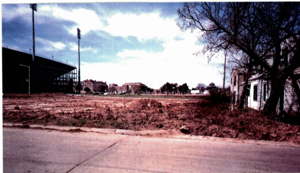
Figure 28. Lot 100 Under Construction, Spring 1989.
