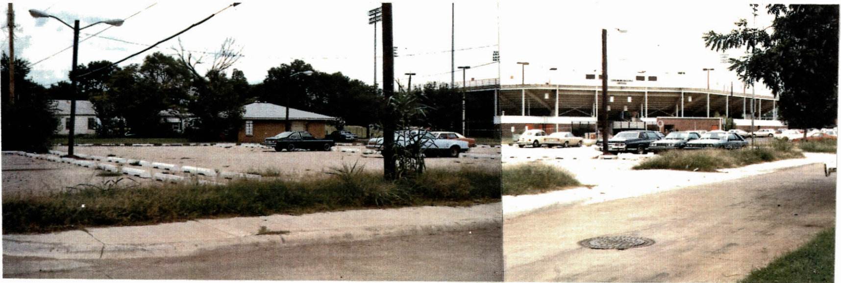
Figure 10. Lot 94 – Temporary Construction Quality Coupled with Lack of Screening.
