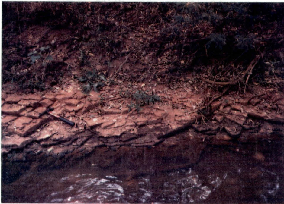
Figure 25. Photograph of Fractured Hennessey Siltstone in Fault Zone.
