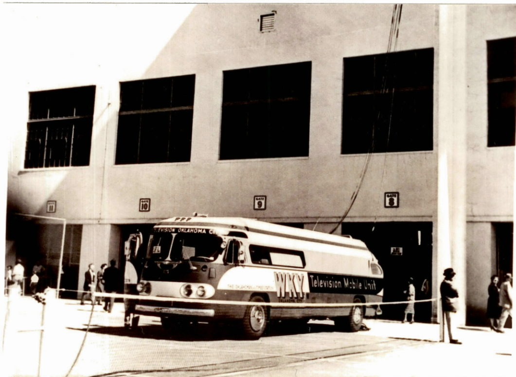
Figure 8. Microwave remote television production truck at University of Oklahoma Football Stadium. Circa 1949. Cables running from truck up side of stadium connect to microwave transmission dish on top of stadium's press box.
