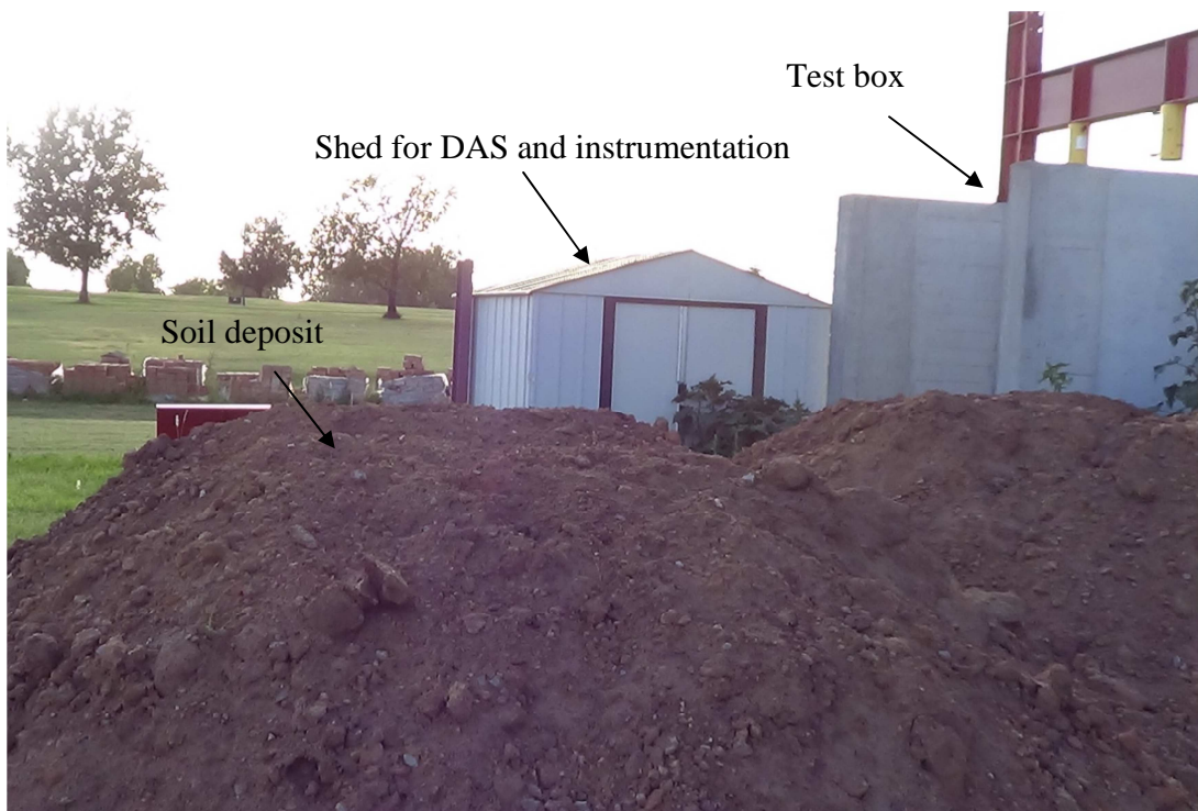
Figure 5.1. Soil deposit at Fears laboratory for full-scale reinforced embankment tests
