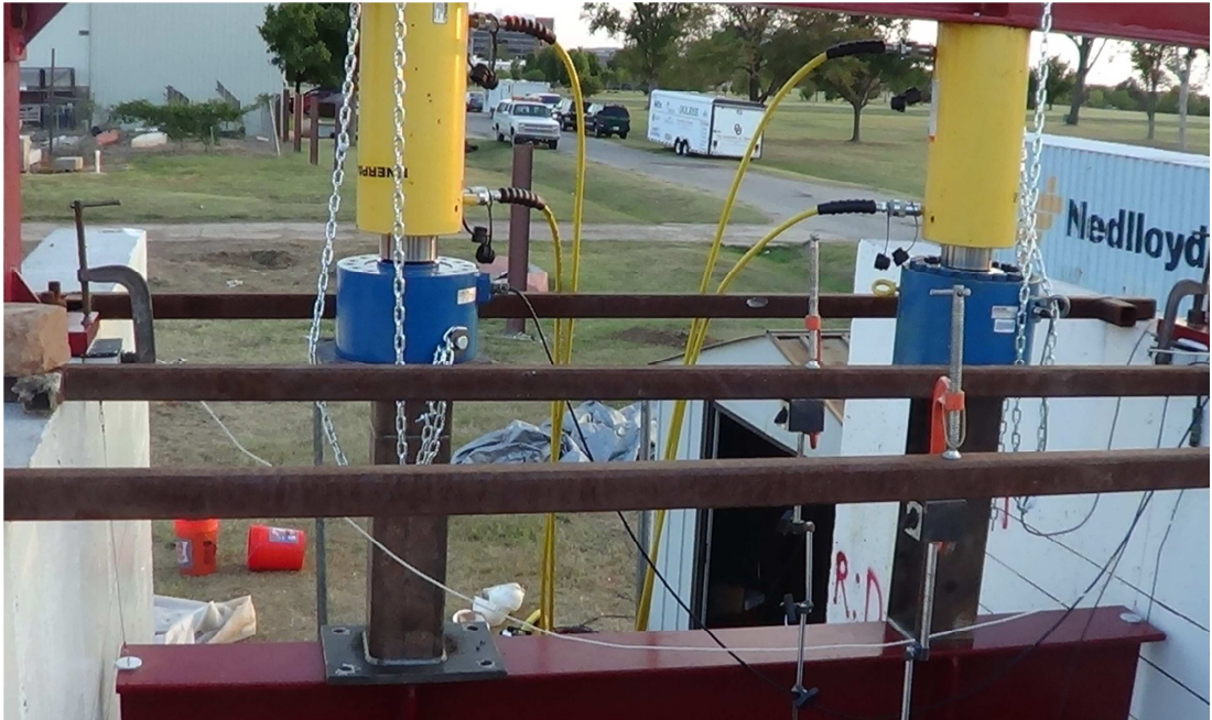
Figure 5.10. Hydraulic cylinders and load cells used for embankment test
