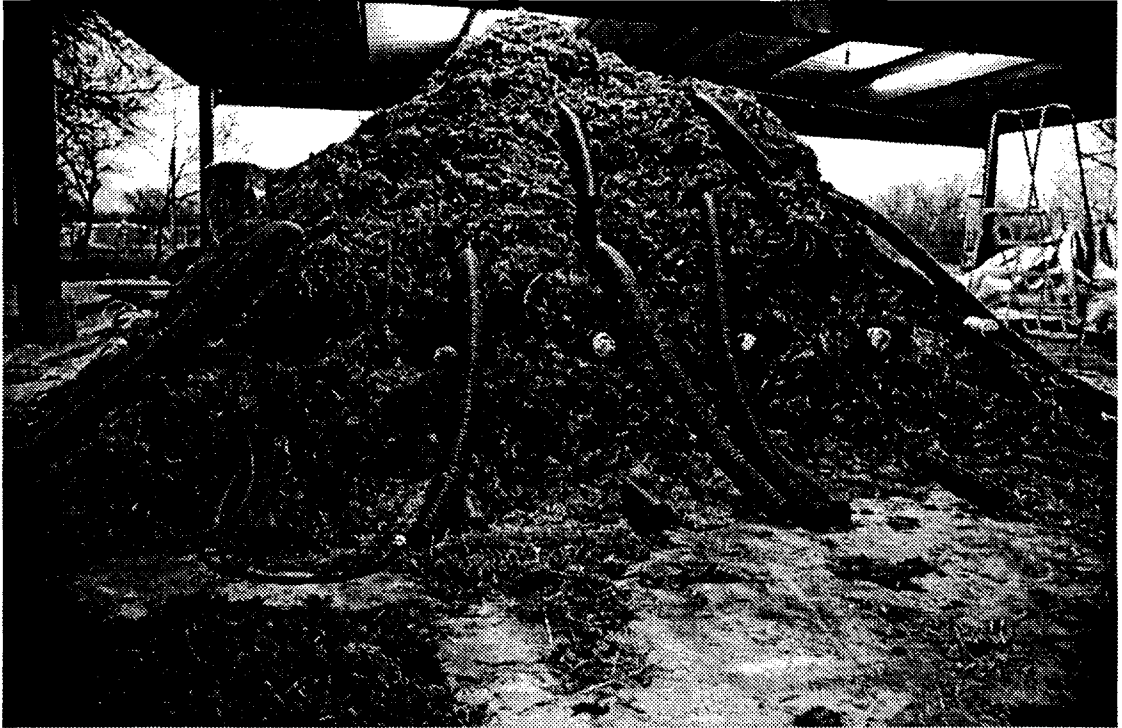
Figure 13. Photo of SP Near Completion with Forced-Air Tubing Capped Off
