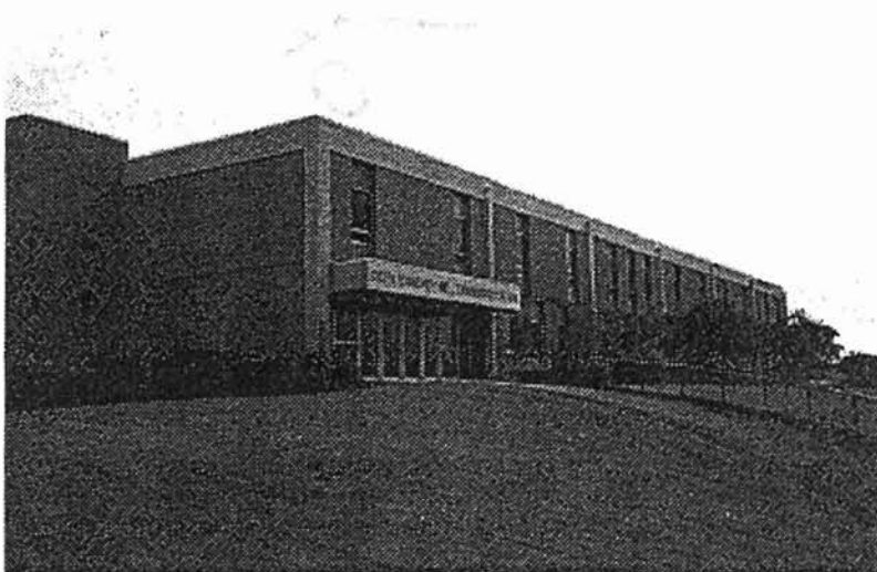
Department of Transportation Building
