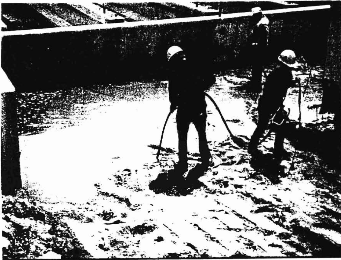
Figure 15. Flooding and Vibration at C2
