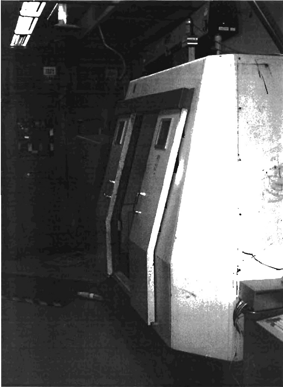
Figure 18 View of power supply enclosure, laser enclosure, and CNC station housing.
