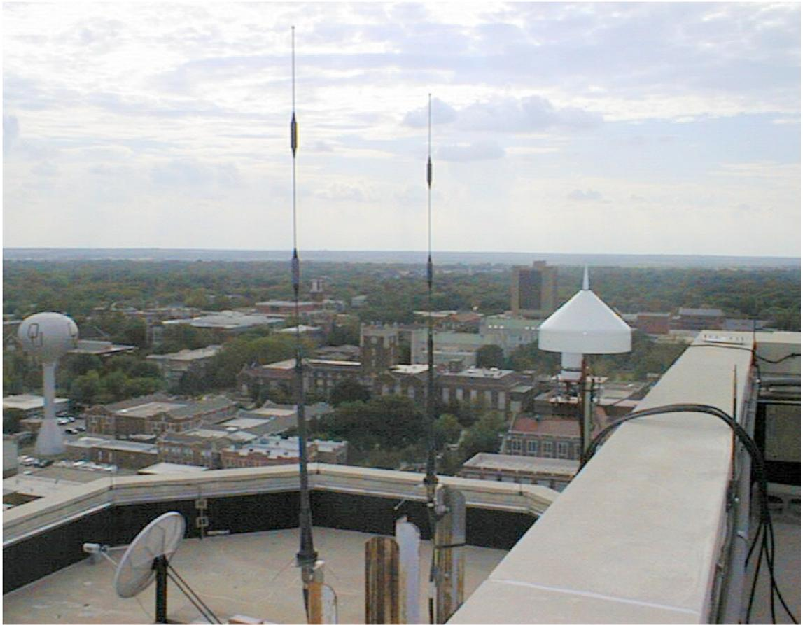
Figure I.4: GPS Reference Antenna on top of the Sarkey Energy Center at the University of Oklahoma.
