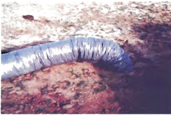
Figure 2-15. Round Duct Insulation Covering Pipe
