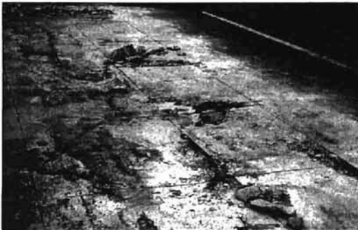
2. Full-depth sawed pavement for removal.
