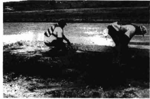
5. Drilling holes for transverse steel
