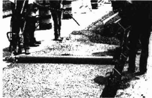
14. Internal vibrator and levelling roller to consolidate and level concrete.
