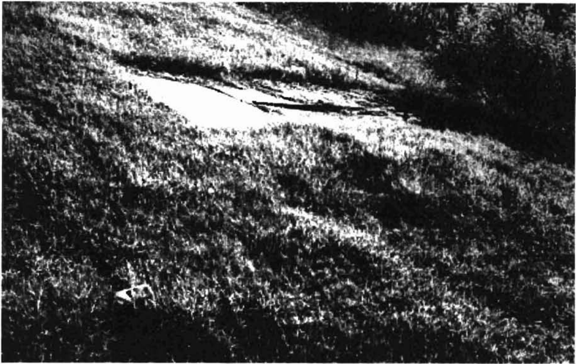
Figure A37. Exit of pavement underdrain northbound.
