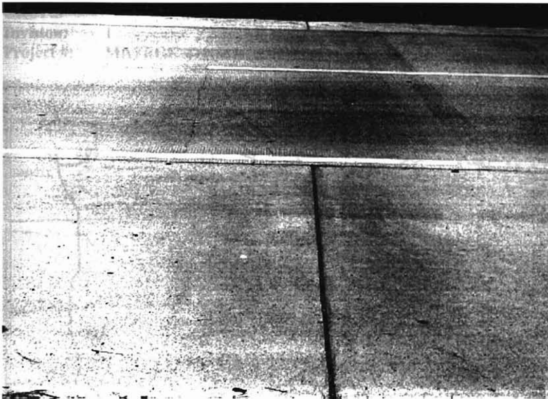
Figure A5. Typical view of SAP-51(392) southbound
