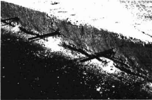
11. Close view of transverse steel installed.
