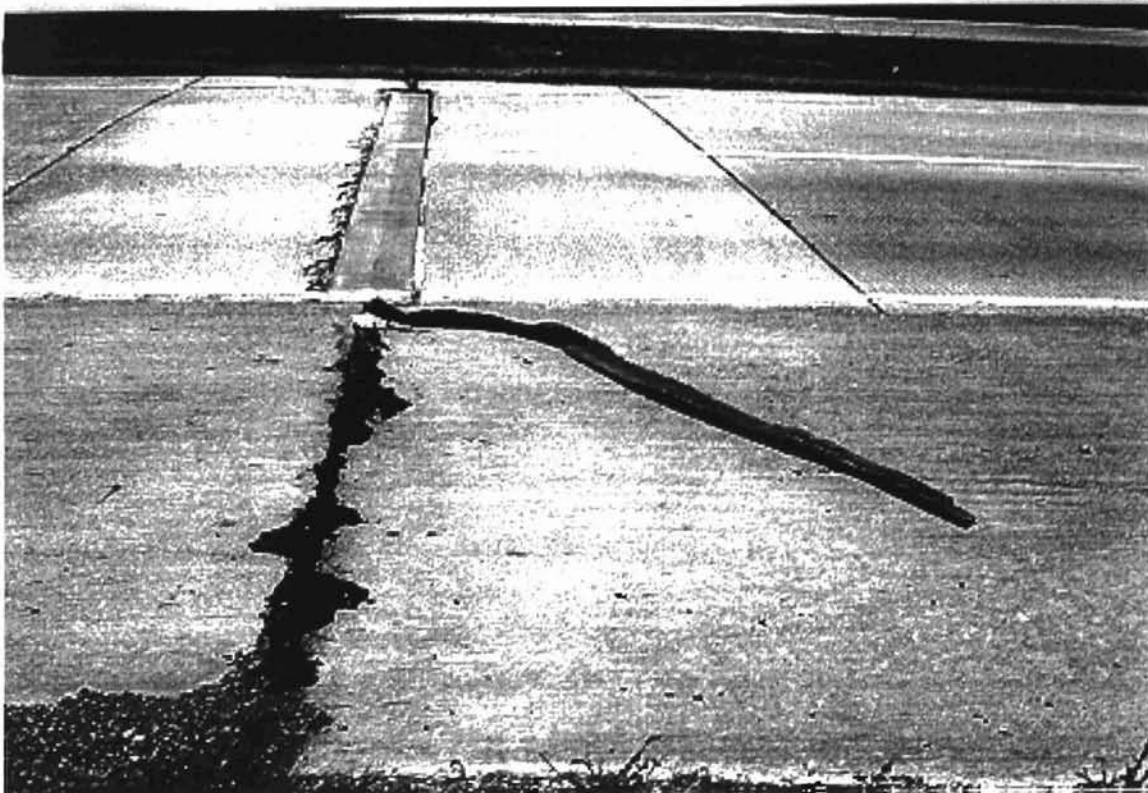
Figure A53. Structural steel beam in terminal joints of F-299(99). Extruded joint filler on shoulder
