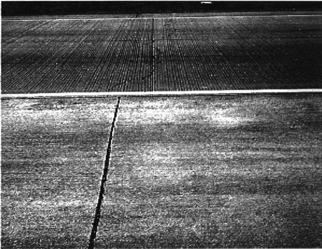
Figure A47. Typical shoulder and pavement condition of F-299(45) southbound.
