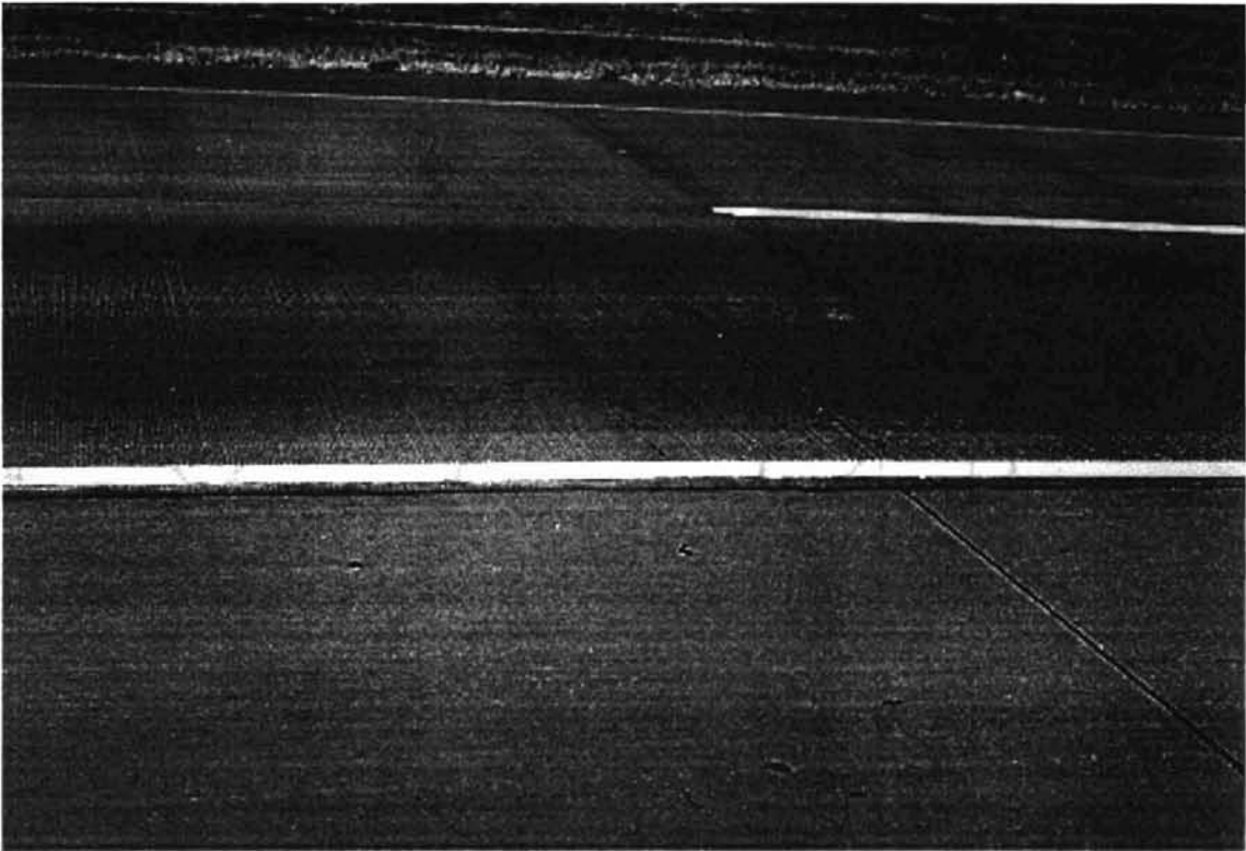
Figure A49. Typical pavement condition on F-299(35) northbound.
