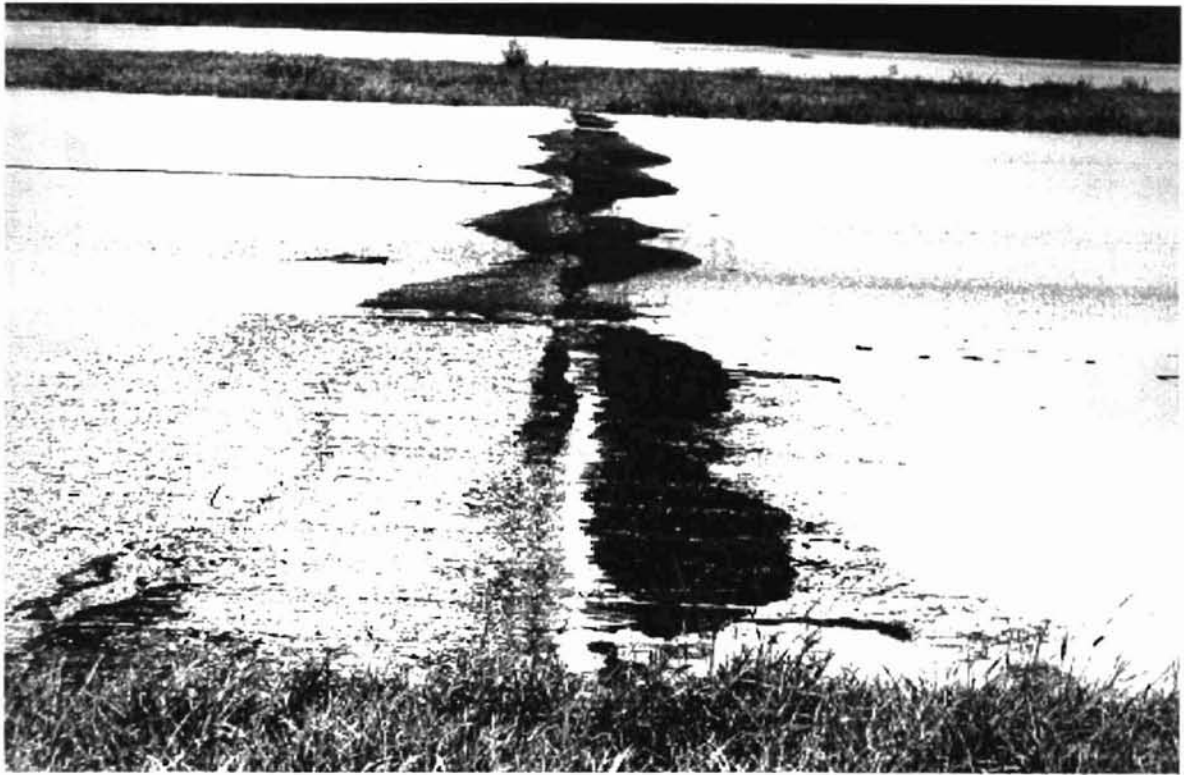
Figure A120. Patch at joint of CRC and asphalt pavements.
