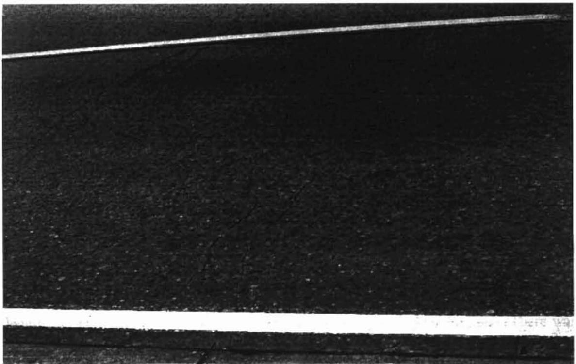
Figure A59. Typical condition of MAF-235(009) westbound.
