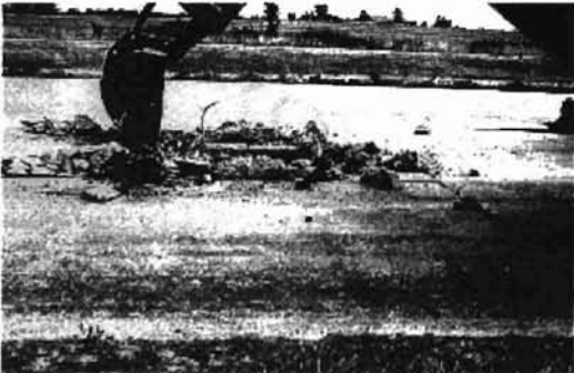
3. Removal of sawed sections.
