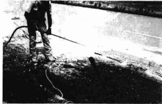
6. Blowing out dust from holes.
