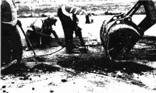
10. Tapping transverse steel into epoxy-injected holes.
