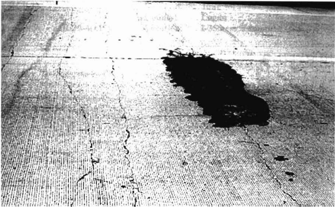
Figure A61. Repair of punchout on I-40 using asphalt concrete patching.
