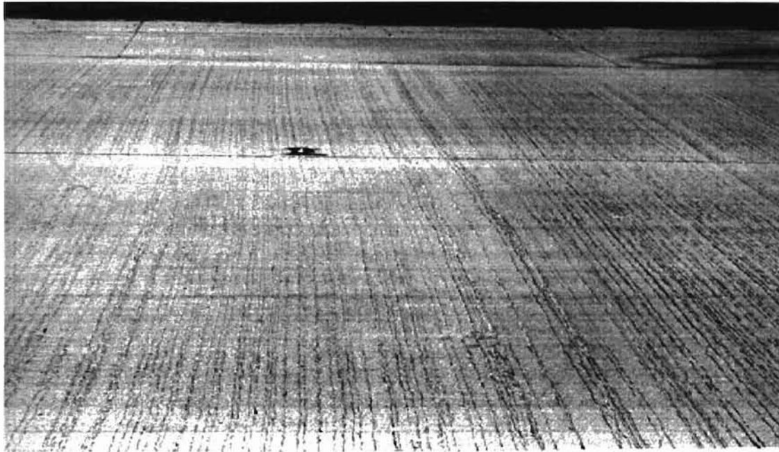
Figure A19. Typical view of CRC on STP-11B(334)
