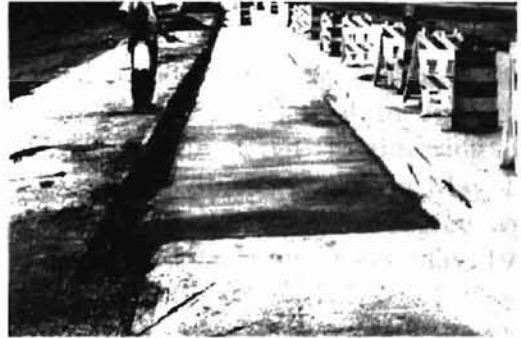
15. Curing concrete.
