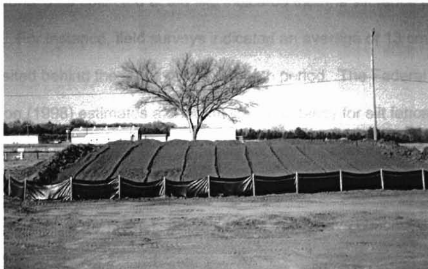
Figure 4: View of the silt fence field site.
