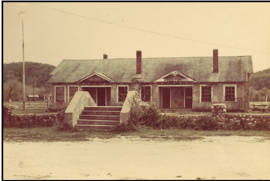
Source: Adair County Historical and Genealogical Association, Stilwell, Oklahoma. Photograph by J.L. Hallford. WPA flagstone veneer added to frame building.
