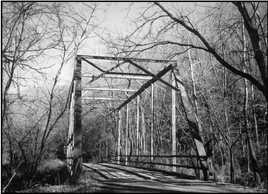
Figure 1.1. Bridge spanning Ballard Creek east of Watts, Oklahoma and constructed through the efforts of FERA and CWA. Undated photograph. Bridge no longer extant.
