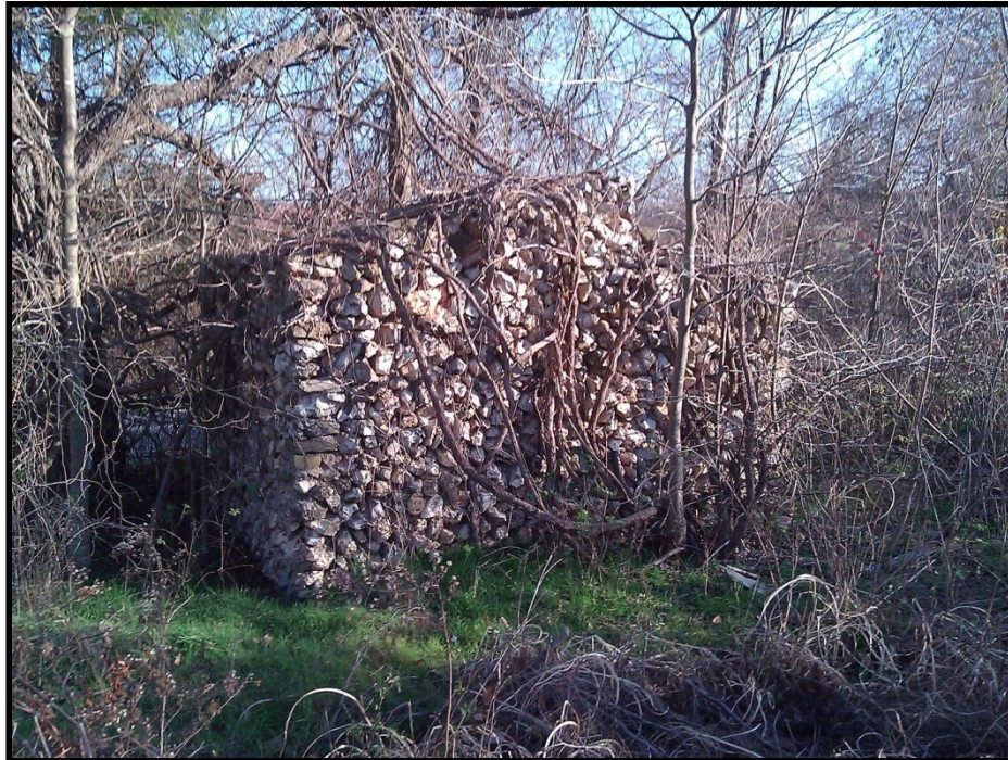
Remnants of stone privy constructed by WPA.
