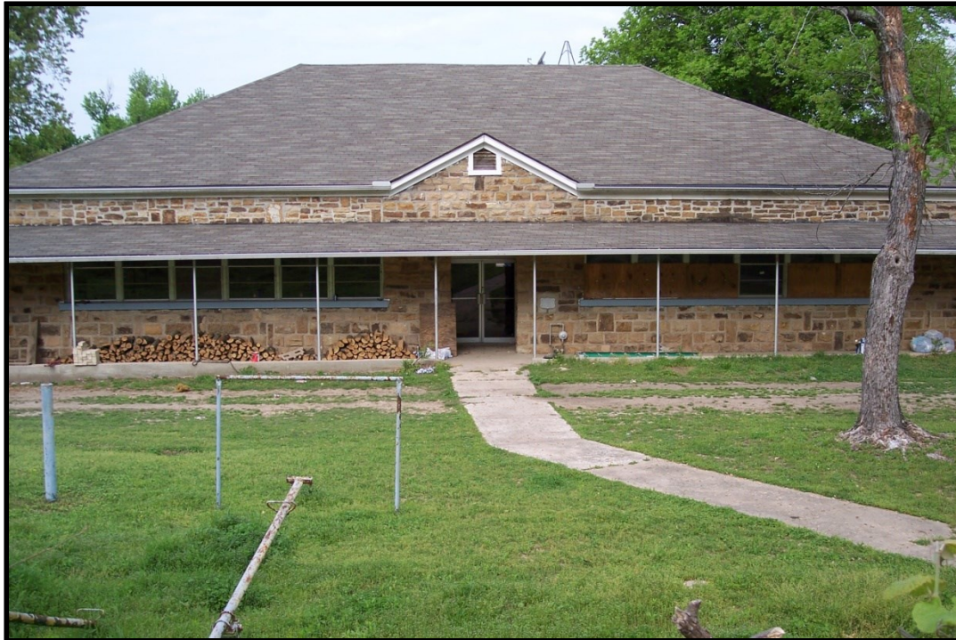
Figure 2.6. Modern, four-room, native-stone school building constructed at Christie by WPA labor in 1939.
