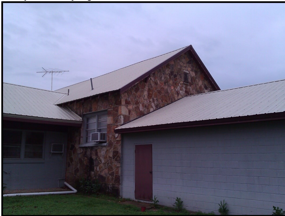
Original WPA rock building and later additions to the north and east.
