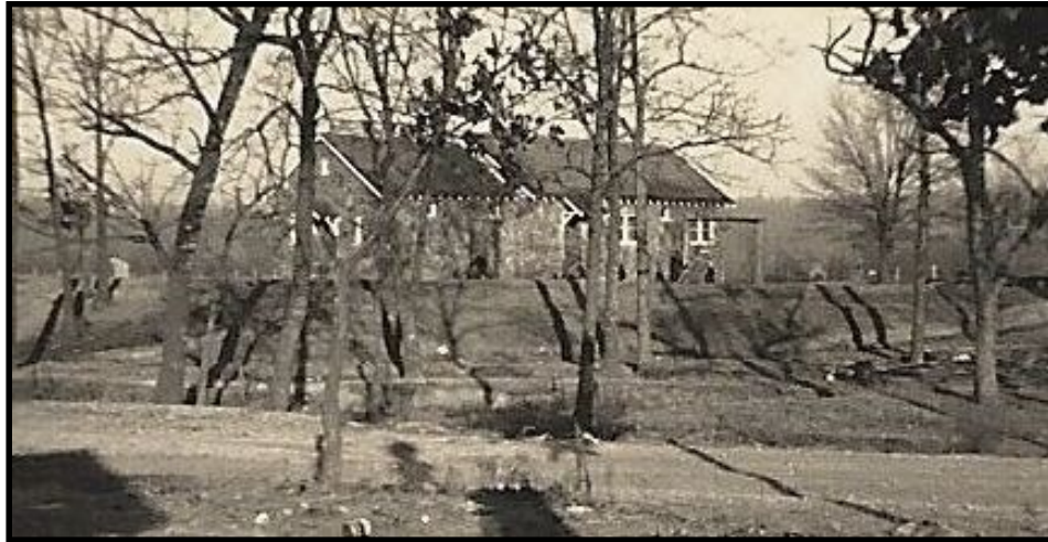
Source: Adair County Historical and Genealogical Association, Stilwell, Oklahoma. WPA two-room flagstone school building. Note the original bi-level roof.
