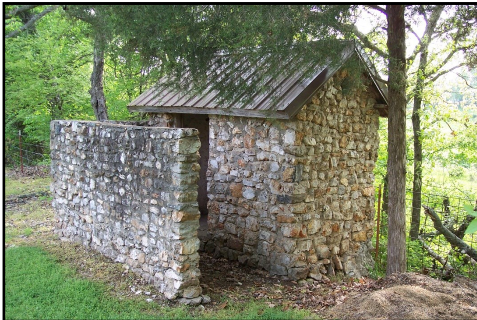
Clearfork School. WPA Toilet.
