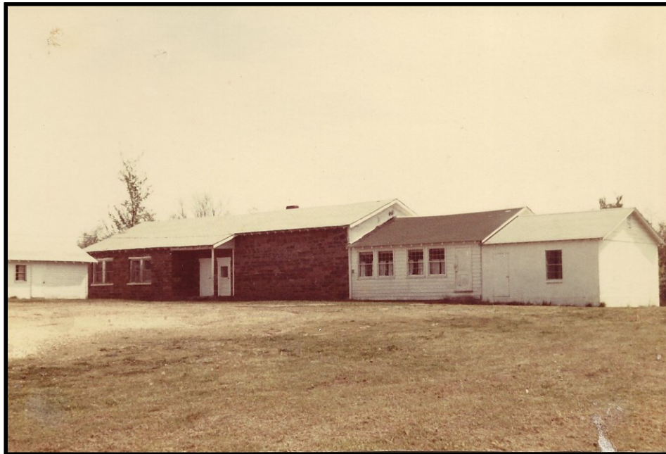
Source: Adair County Historical and Genealogical Association, Stilwell, Oklahoma. Photograph by J.L. Hallford. Photograph depicts additions made to building to the west and south.
