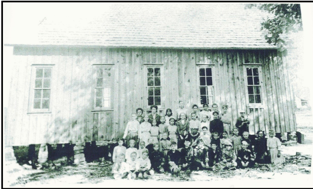
Figure 2.5. Christie School building of frame construction prior to New Deal.
