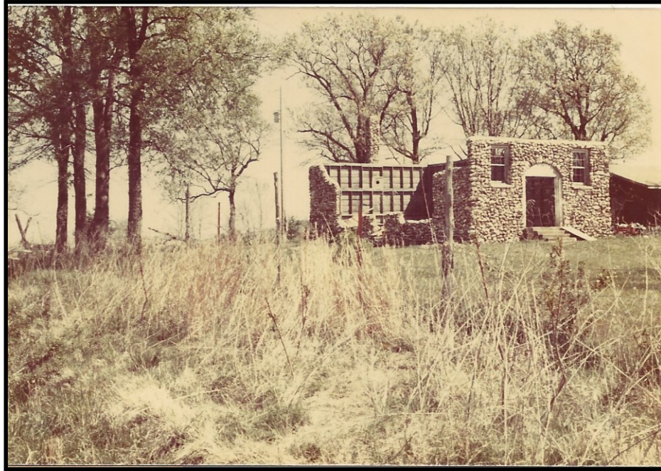
Source: Adair County Historical and Genealogical Association, Stilwell, Oklahoma. Photograph by J.L. Hallford. Remains of Union Hill School following fire.
