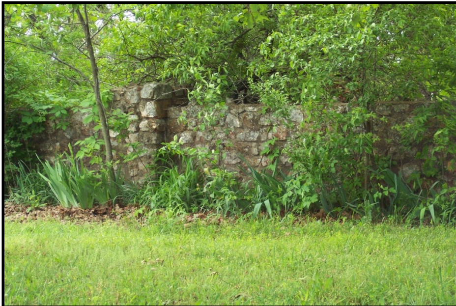
Rock wall built by WPA on school grounds.
