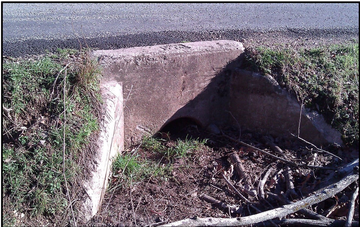
Cement culvert constructed in Baron, Oklahoma by WPA labor in 1939.
