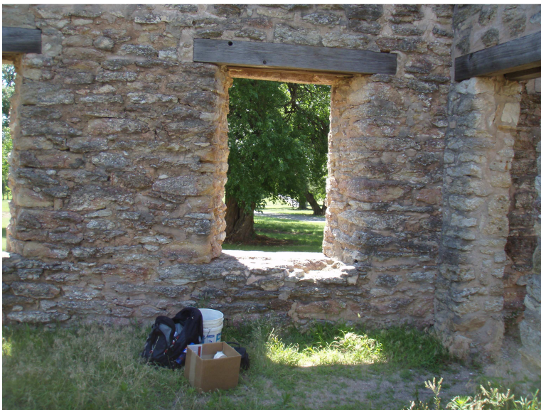
Figure 6. Interior of barracks showing stone work of the 1st reconstruction at Fort Washita.
