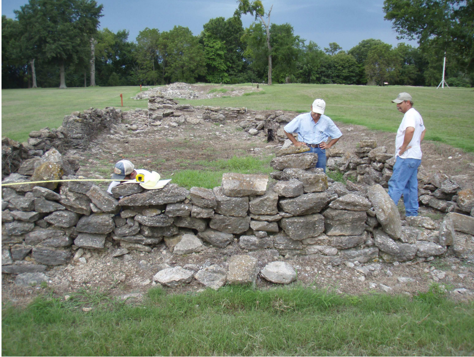
Figure 13. Partially re-constructed barracks wall without pointing at Fort Towson.
