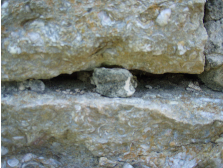
Figure 7. Stone wall constructed of the local limestone. Mortar samples were obtained from the original wall and were 1st generation mortar at Fort Washita.
