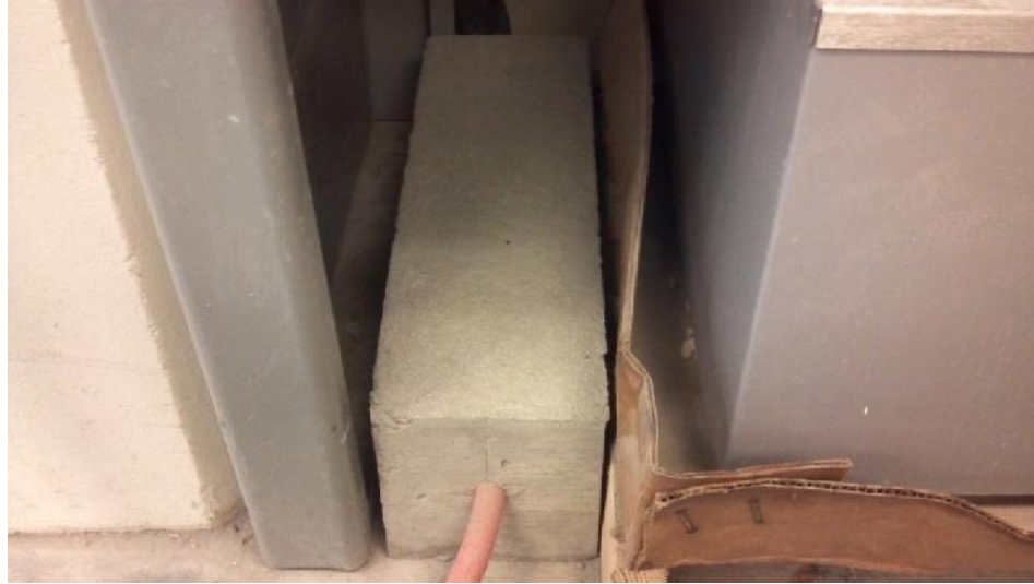
Figure 7: Concrete vibration damper
