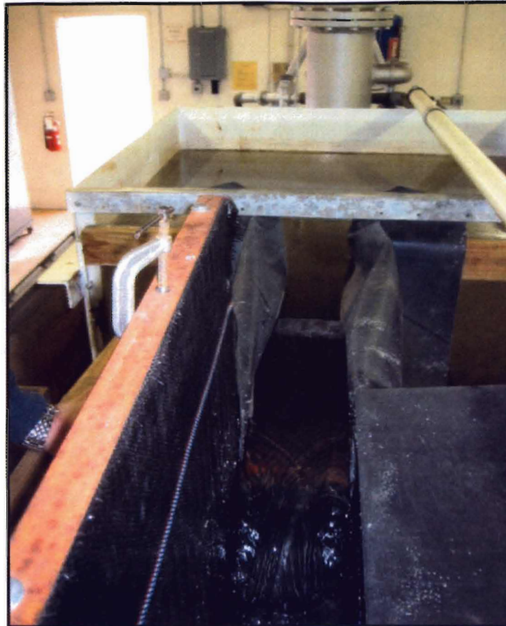
Figure 3.3: Rubber-lined connection of upstream reservoir to inlet of trench
