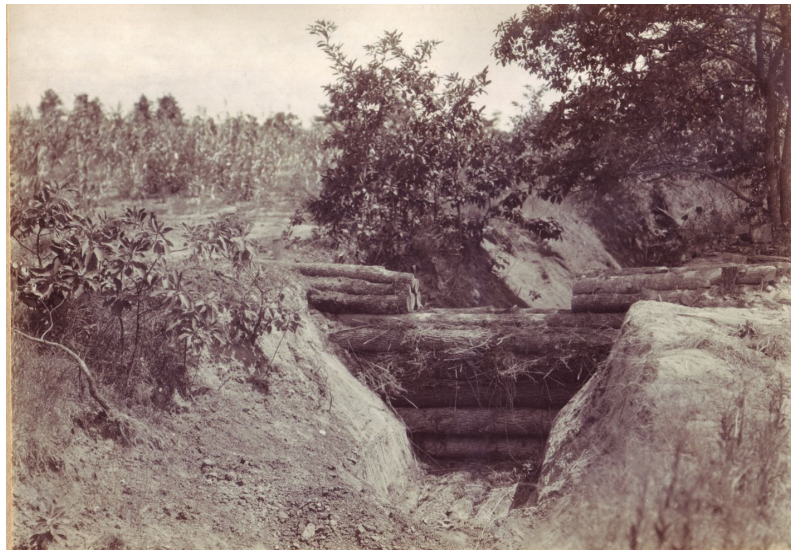
Figure 20. Photo of a check dam made from logs on the soil erosion experiment station at Tyler, Texas, July 21, 1930 (RG 114p, Soil Erosion Experiment Station Photographs, Box 15, National Archives, College Park, MD).
