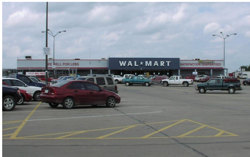
Figure 18: The Old Walmart Building.
