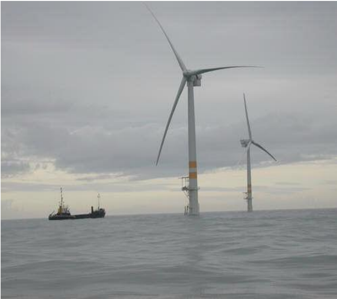
Figure 1. Off-shore 3.6 MW 100m diameter GE turbines off the coast of Arklow, Ireland (Robert Thresher, NREL)
