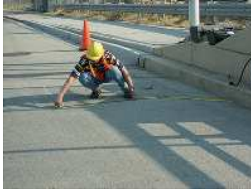
Figure 1.2: A human inspector measures cracks for bridge deck maintenance.
