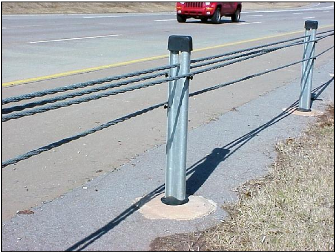
Figure 3: Brifen WRSF on Lake Hefner Parkway (Courtesy of Brifen USA, Inc.)
