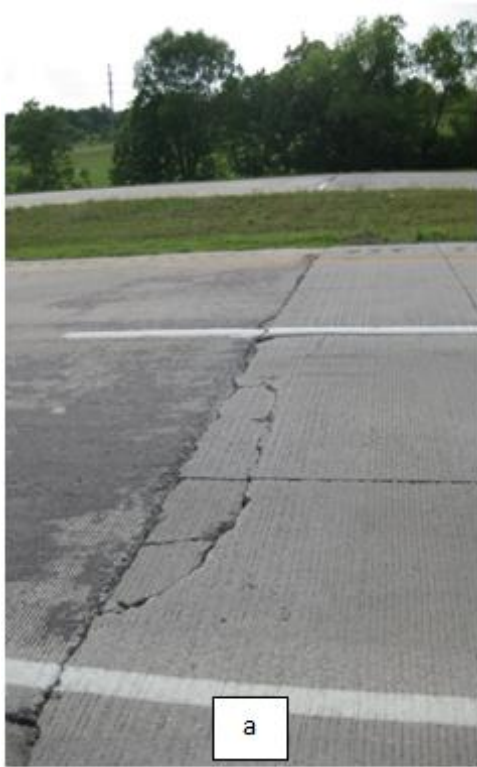
Figure 2.19 – Photo a shows the cracked panels at the junction of the overlay and the existing asphalt pavement. Photo b shows a rare corner crack on the overlay.
