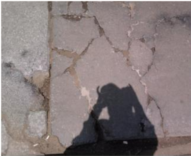
Figure 2.38 - Fines movement in first panels of intersection.
