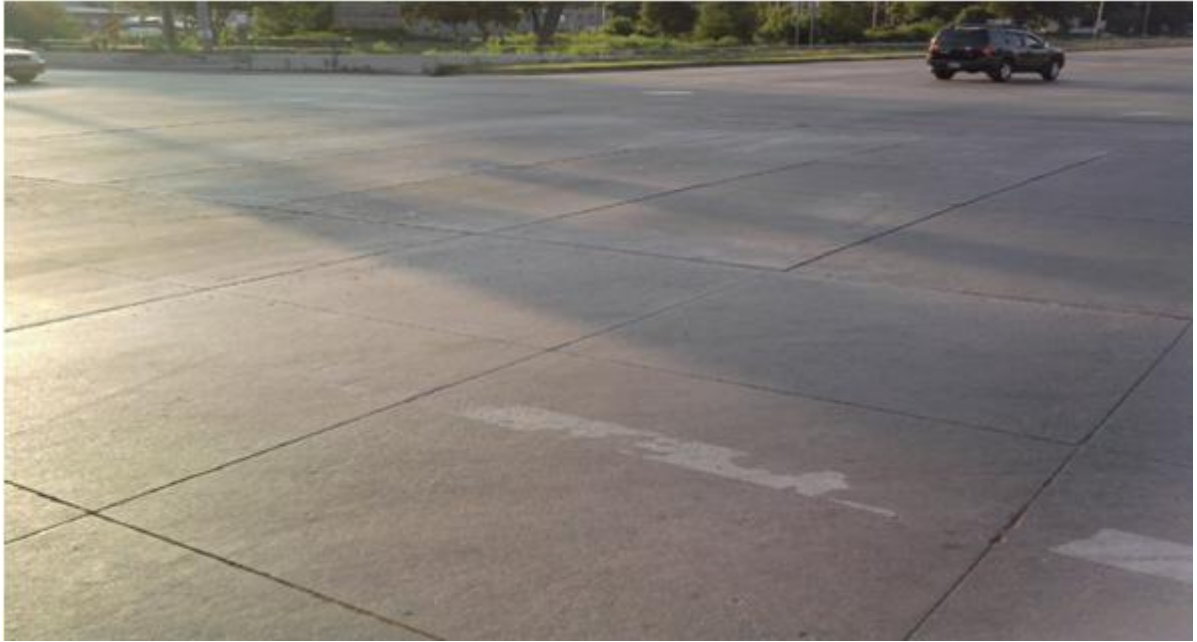
Figure 2.31 - Intersection as seen from the edge of gas station towards north-west.
