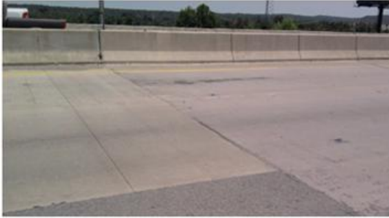
Figure 2.12 – The overlay terminates at a bridge and does not show any distress.
