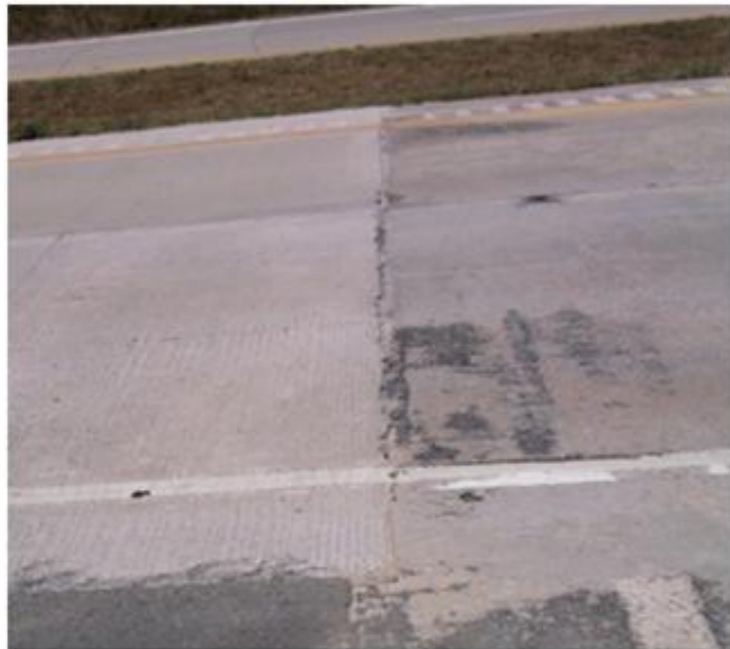
Figure 2.20 – The interface of the overlay and the adjacent pavement is in good condition.
