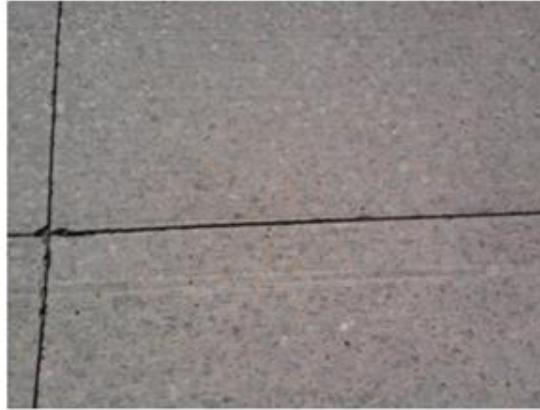
Figure 2.21 – Polishing of the overlay surface.
