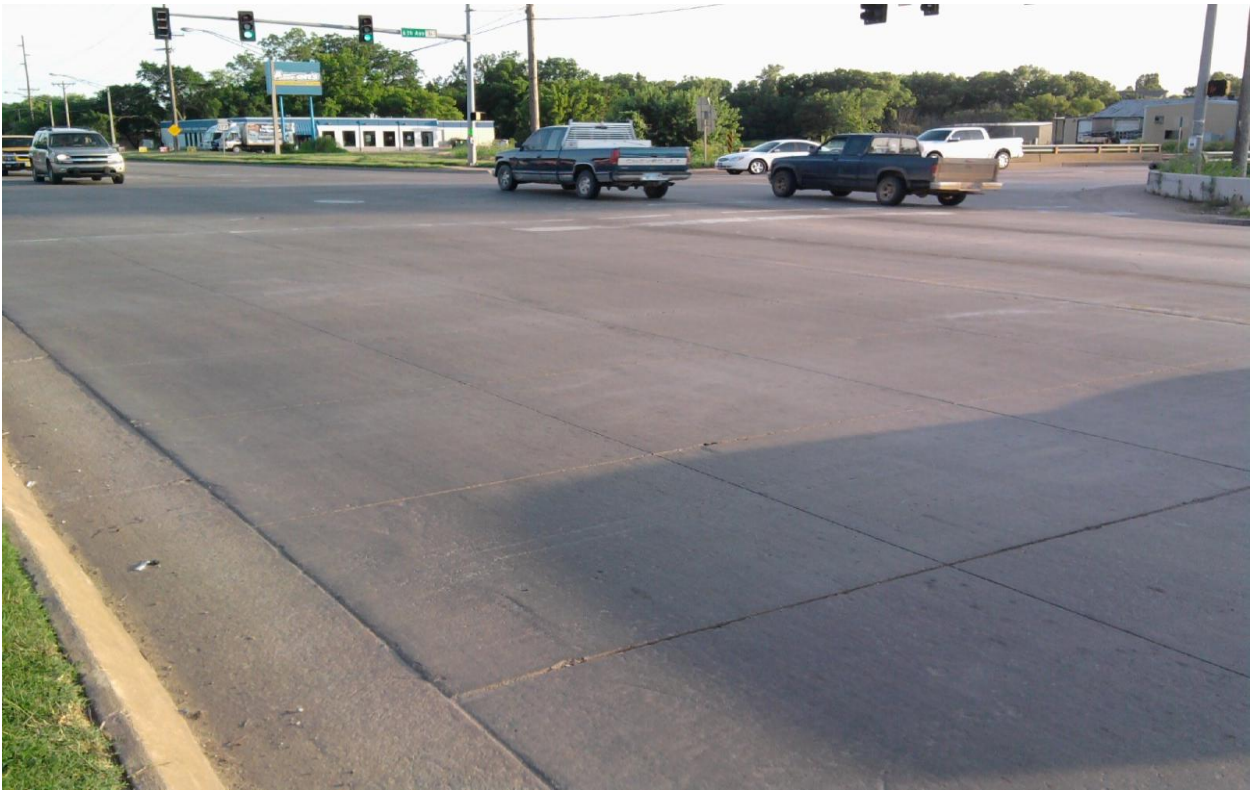
Figure 2.34 - Photo of intersection seen on US 177 towards south-west showing excellent condition of overlay.
