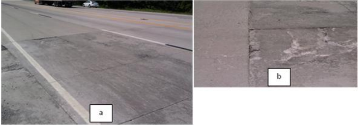
Figure 2.17 – Photo a shows a cracked panel at the start of an overlay. Photo b shows a closer view of that panel.
