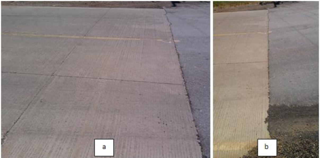
Figure 2.50 - Photos a and b show approach panels in un-distressed condition. Elevation difference between leaving asphalt pavement and approaching concrete panels is almost zero.
