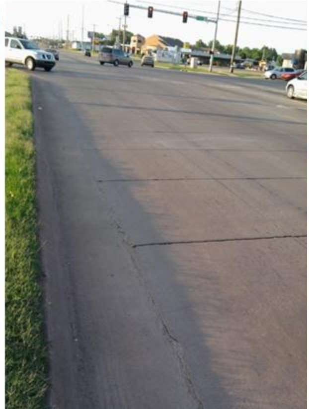
Figure 2.33 - Excellent condition of panels US 177 from the south.
