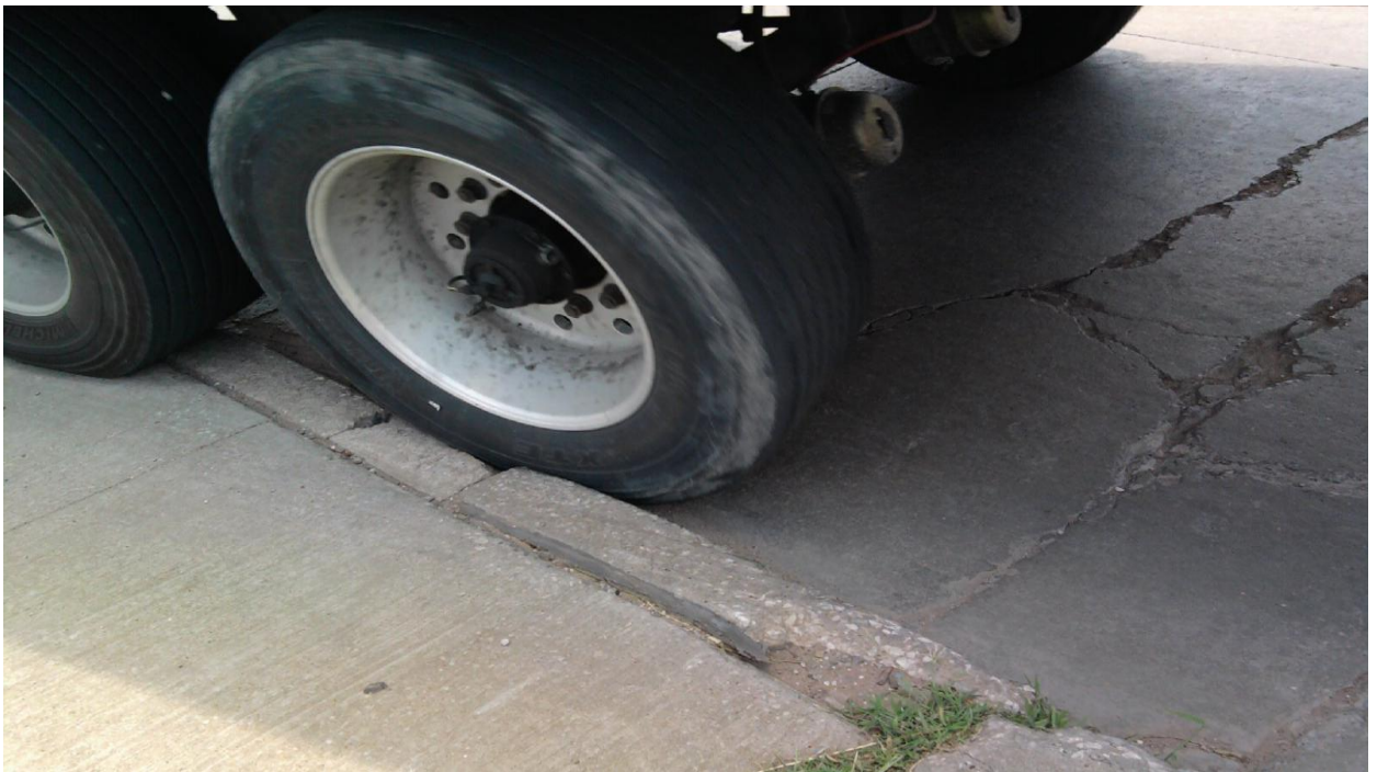
Figure 2.40 - Photo showing the impact loading due to lack of radius of curvature for large trucks.
