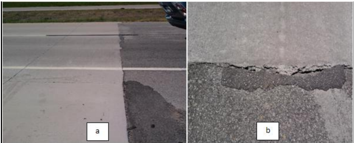
Figure 2.18 - Photo a shows the end of the overlay. The asphalt pavement looks good where it starts. But there is a small amount of distress initiation as shown in photo b.
