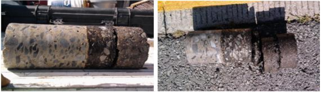
Figure 2.26 - Cores extracted on the oldest McAlester Overlay.
