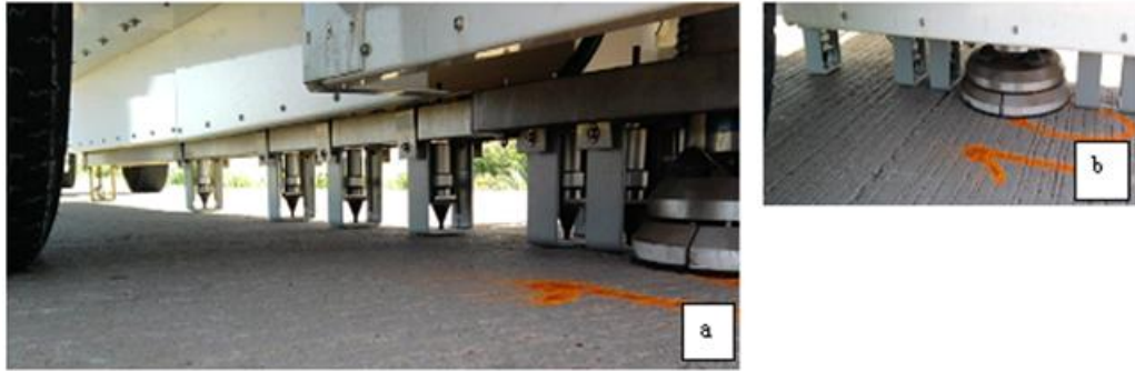
Figure 2.3 – The photos show the layout of the FWD and sensors on the whitetopping.
