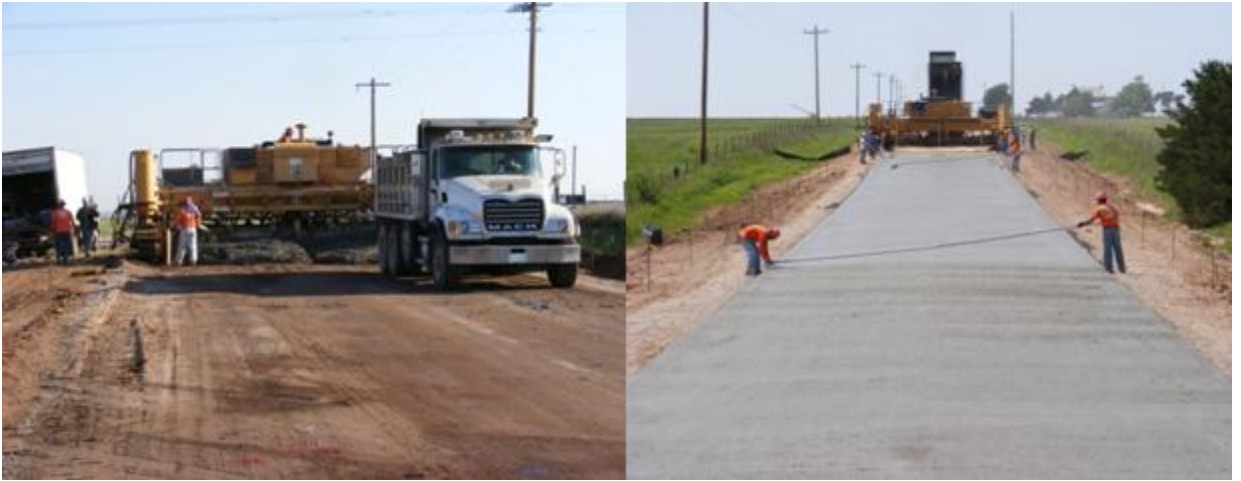
Figure 2.48 - Photos show the construction of the overlay.
