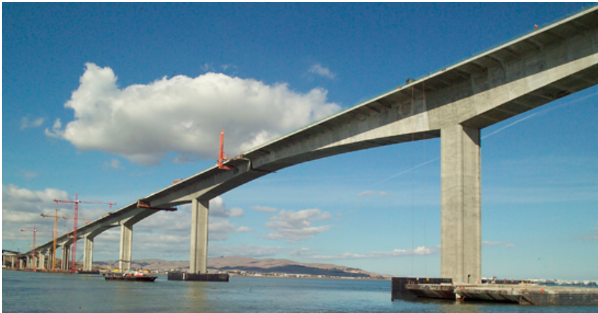
Fig. 3.1. Picture of the New Benicia Bridge (Murugesh, 2008).
