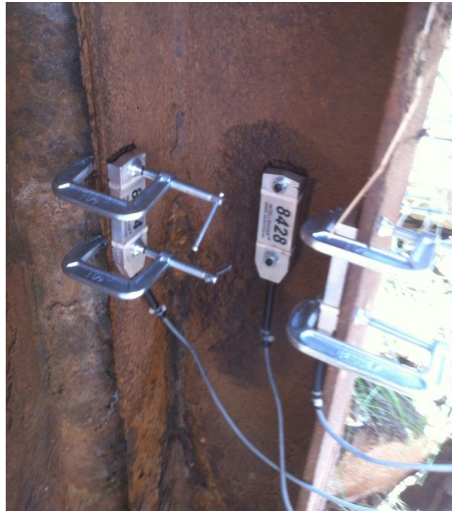
Figure 3.3 Strain Transducers Installed on H-Pile
