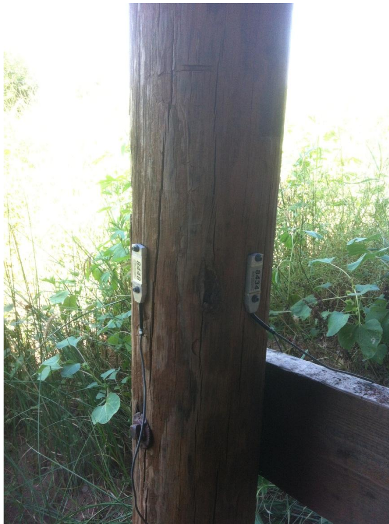
Figure 3.17 Pile N1 and Attached Strain Sensors
