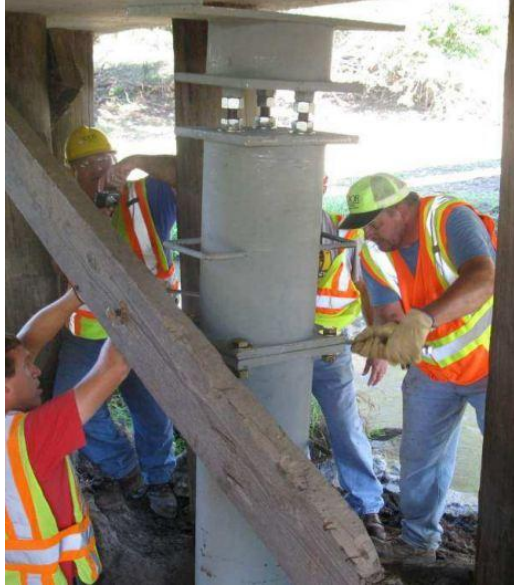
Figure 2.8 Installing the Splice
