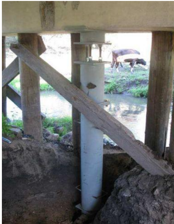
Figure 2.8 Installing the Splice
