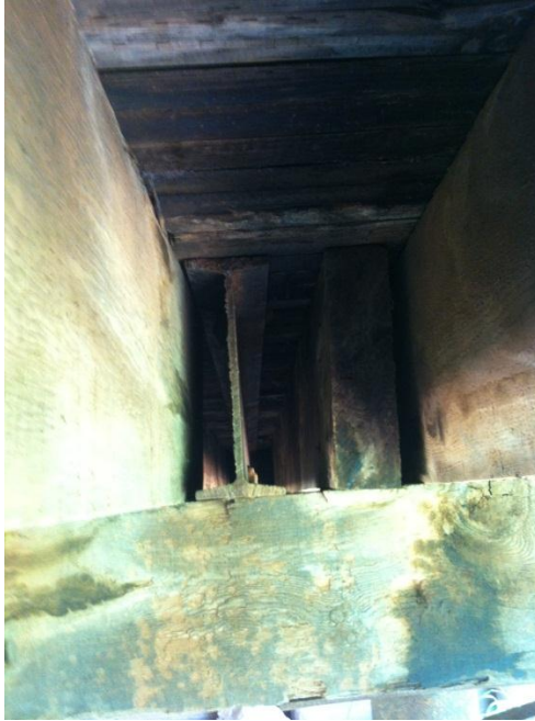
Figure 3.10 W-Shape Acting as a Replacement Timber Beam
