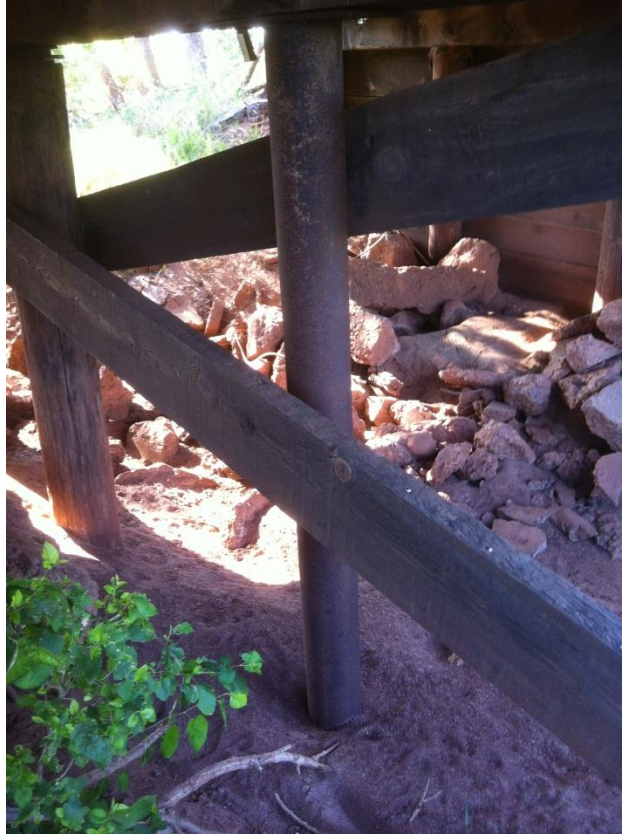
Figure 3.11 Installed Steel Splice
