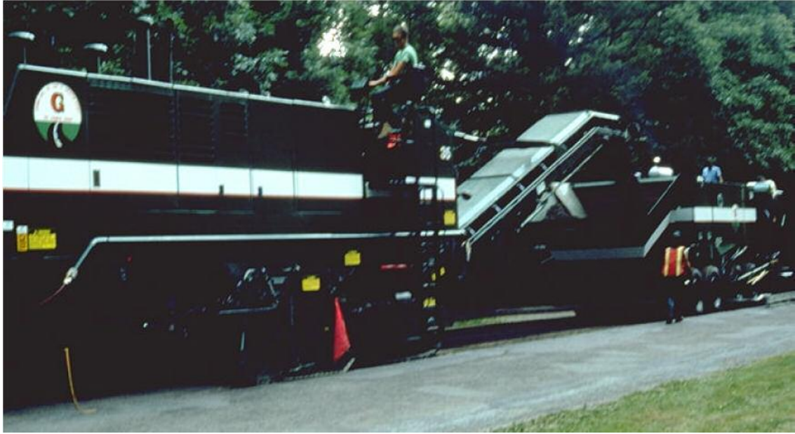
FIGURE 2-6 A Paver Mixer Two-Unit CIR Train.
