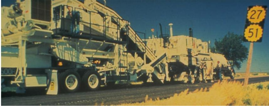
FIGURE 2-8 Portable Crusher Attached to a Cold Milling Machine [10].
