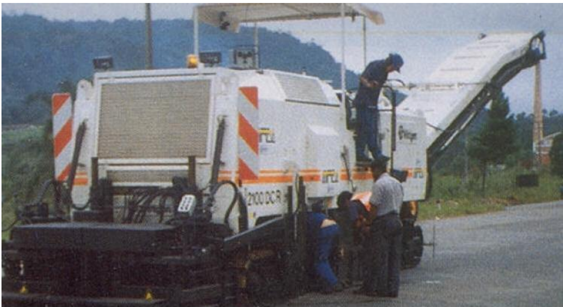
FIGURE 2-9 Cold Milling Machine [10].
