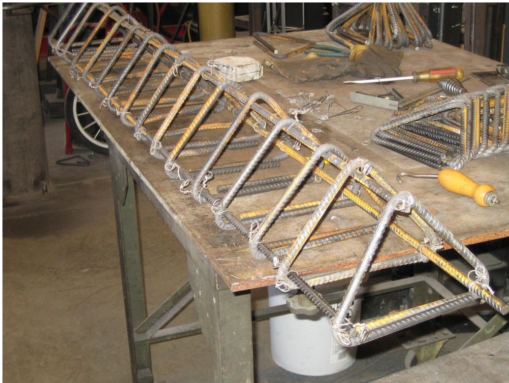
Figure 3.4: Bottom bulb confining reinforcement
