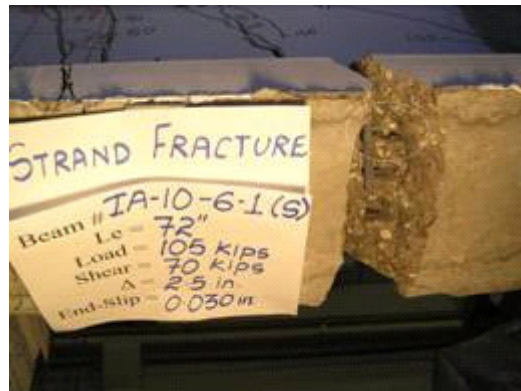
Figure 4.7: Photo showing the fractured strand (Test : IA-10-6-1-S)
