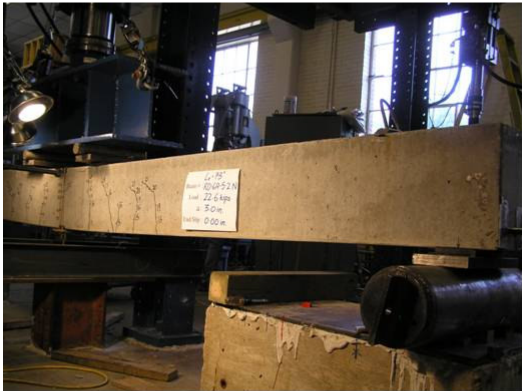
Cracking pattern for Beam RD-6A-5-2 being loaded at North end
