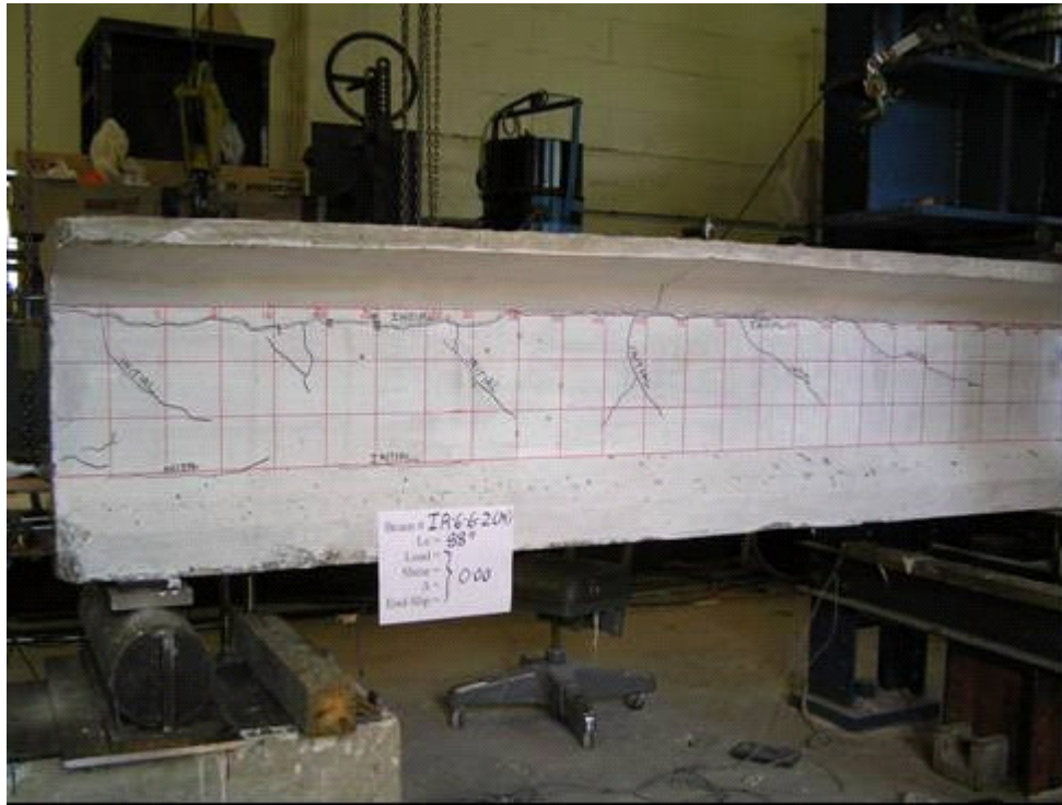
Figure 4.14: Photo showing the cracks present on the beam IA-6-6-2 before starting the test.
