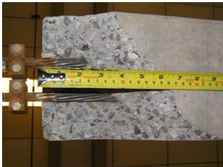
Damage caused during transportation at the North end (bottom).
