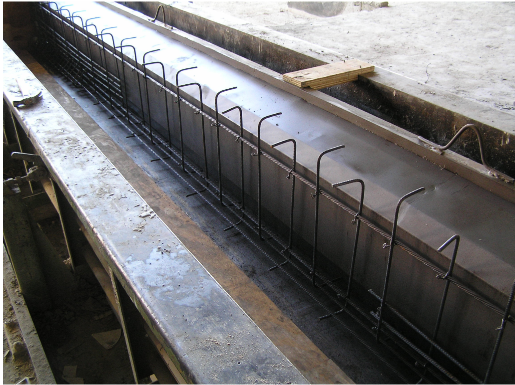
Figure 3.3: Arrangement of stirrups for I-shaped beams
