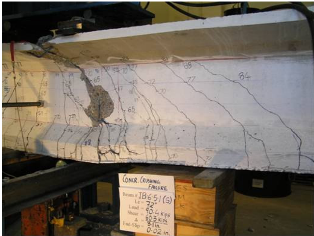
Photo of the crushed region of beam IB-6-5-1 (South end test)
