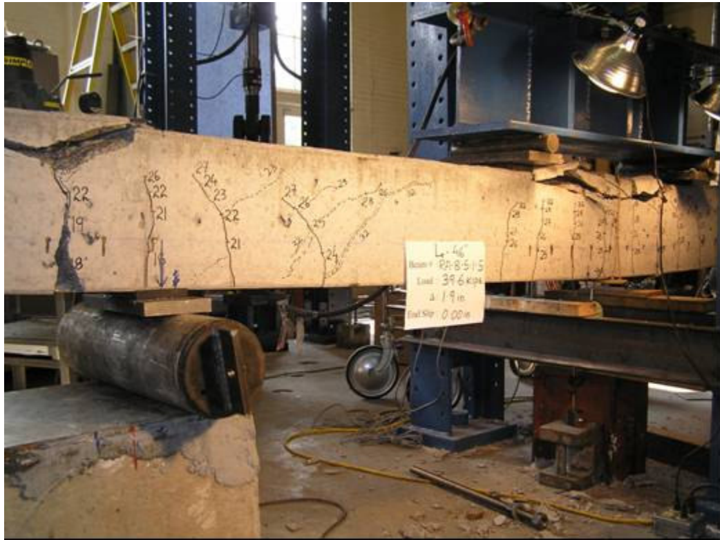
Cracking pattern at the North Support for Beam RA-8-5-1 (South side being tested)
