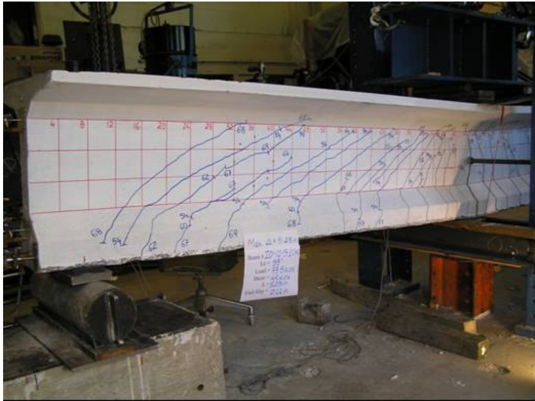
Photo of North end of beam ID-10-5-1 showing the cracking pattern at the maximum load
