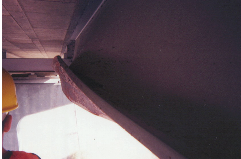
Figure 1.1: Deformation of Flange Due to Impact, < http://www.steelstraightening.com/arizona.htm >
