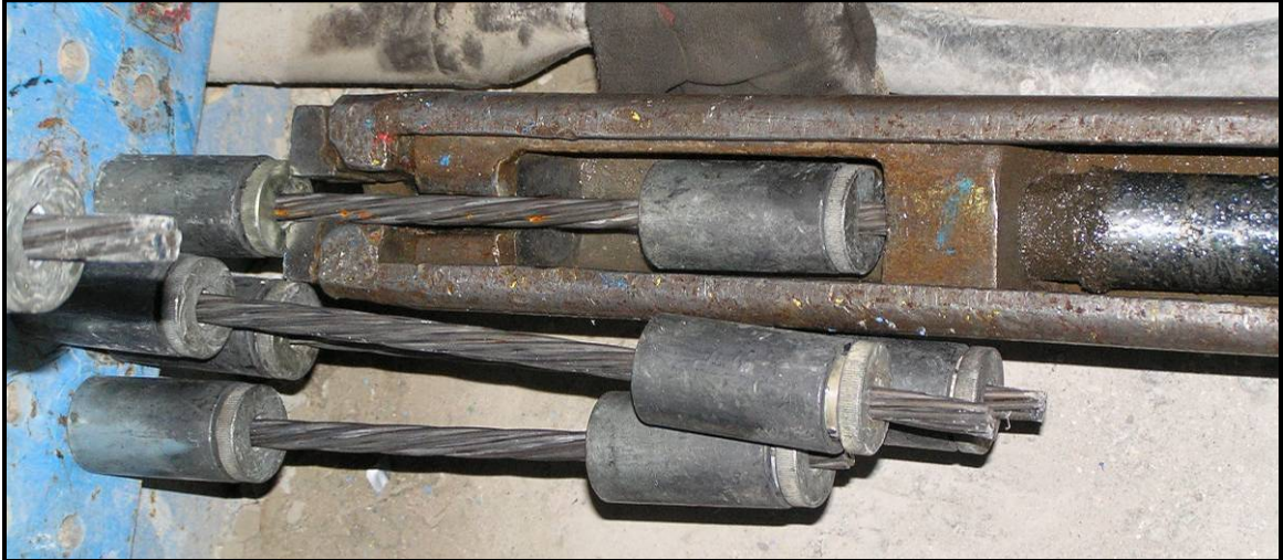
Figure 5.6: Prestressing the strands using hydraulic ram
