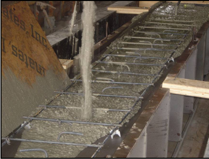
Figure 5.7: Vibrating concrete on I-beams
