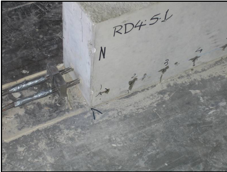
Figure 5.26: Reference position before flame cutting for RD4-5-1
