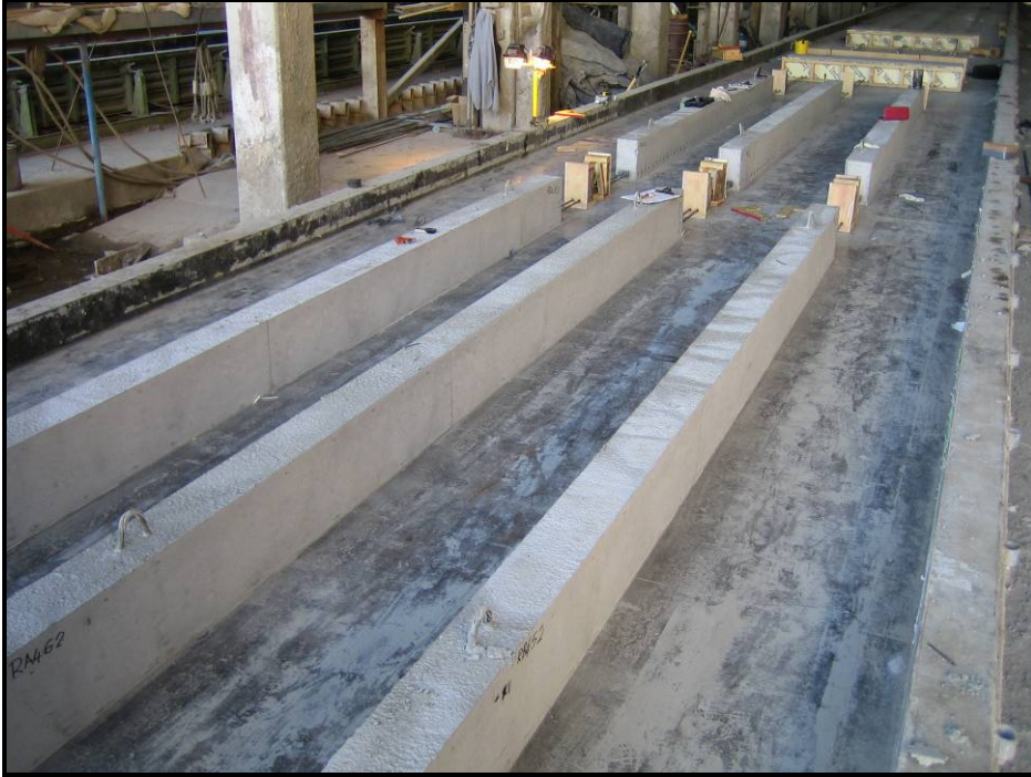
Figure 5.3: Fabrication of Rectangular beams
