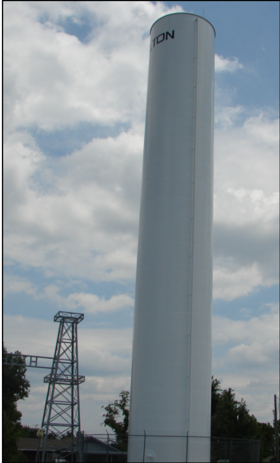
Figure 3: Picture of the 600,000 gallon standpipe in the town.
