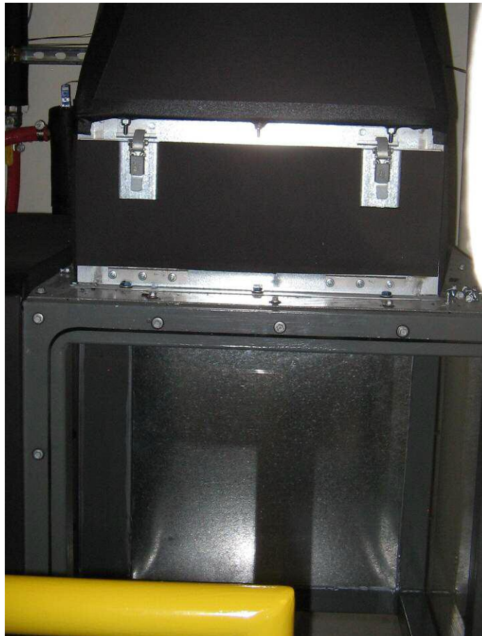
Figure D-3 Air filter housing before main cooling coil
