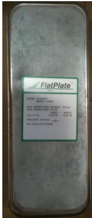
Figure 1-1. Brazed plate heat exchanger
