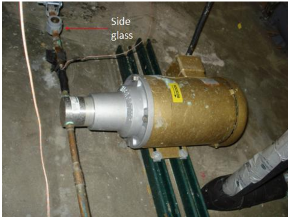
Figure 3-13. Refrigerant Pump
