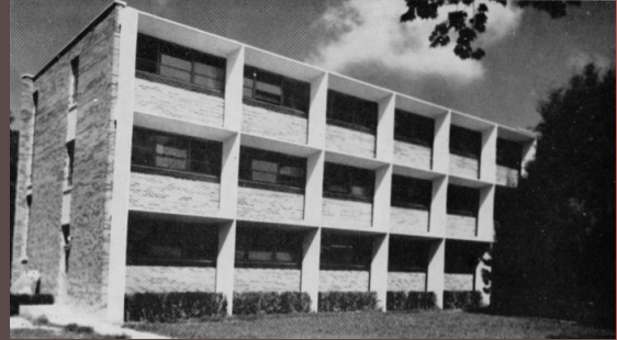
FIGURE 2.6: ORIGINAL COLLINGS HALL FACADE
