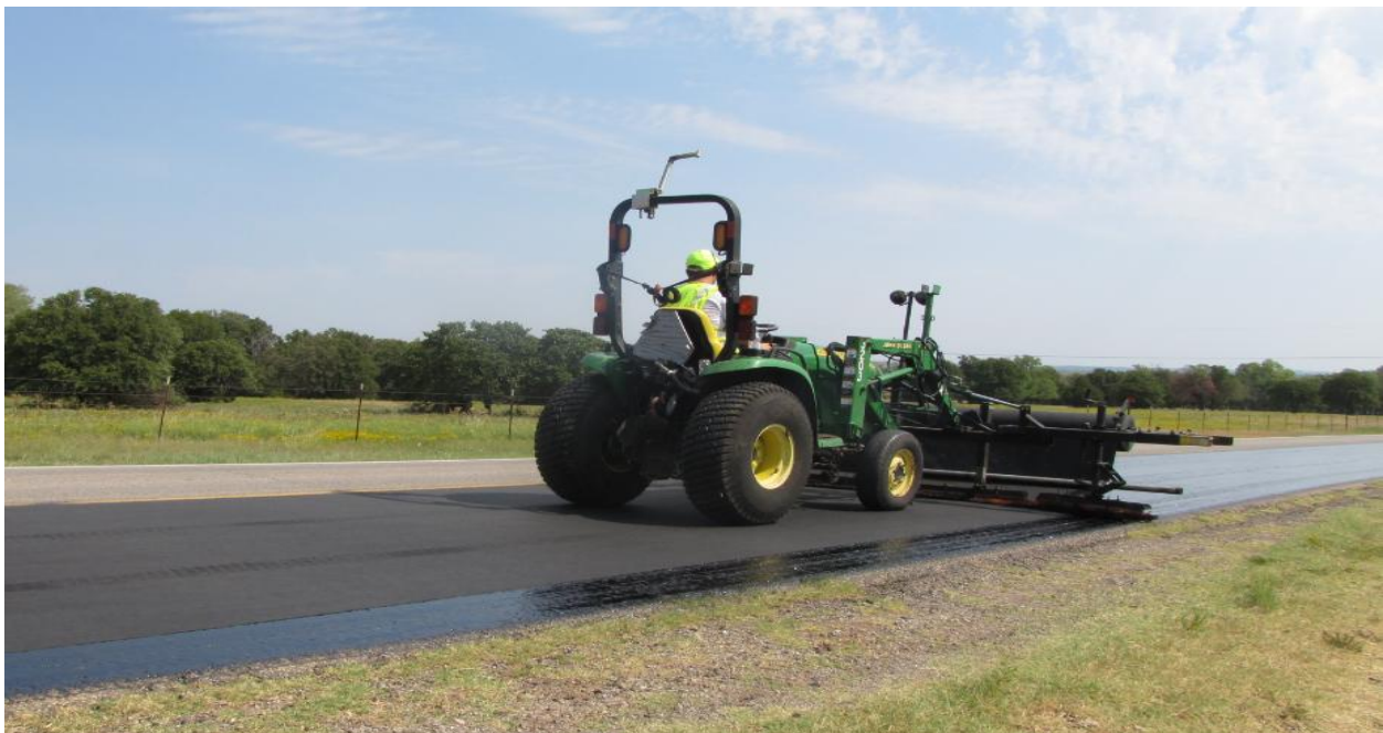
Figure 4.8 Geosynthetic (Paving) Fabric Being Installed in Test Sections
