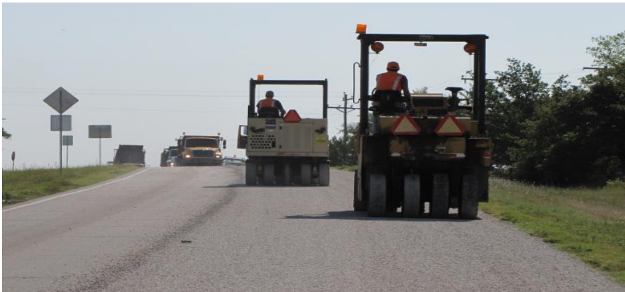
Figure 6.7 Chip Seal Rolling Operation
