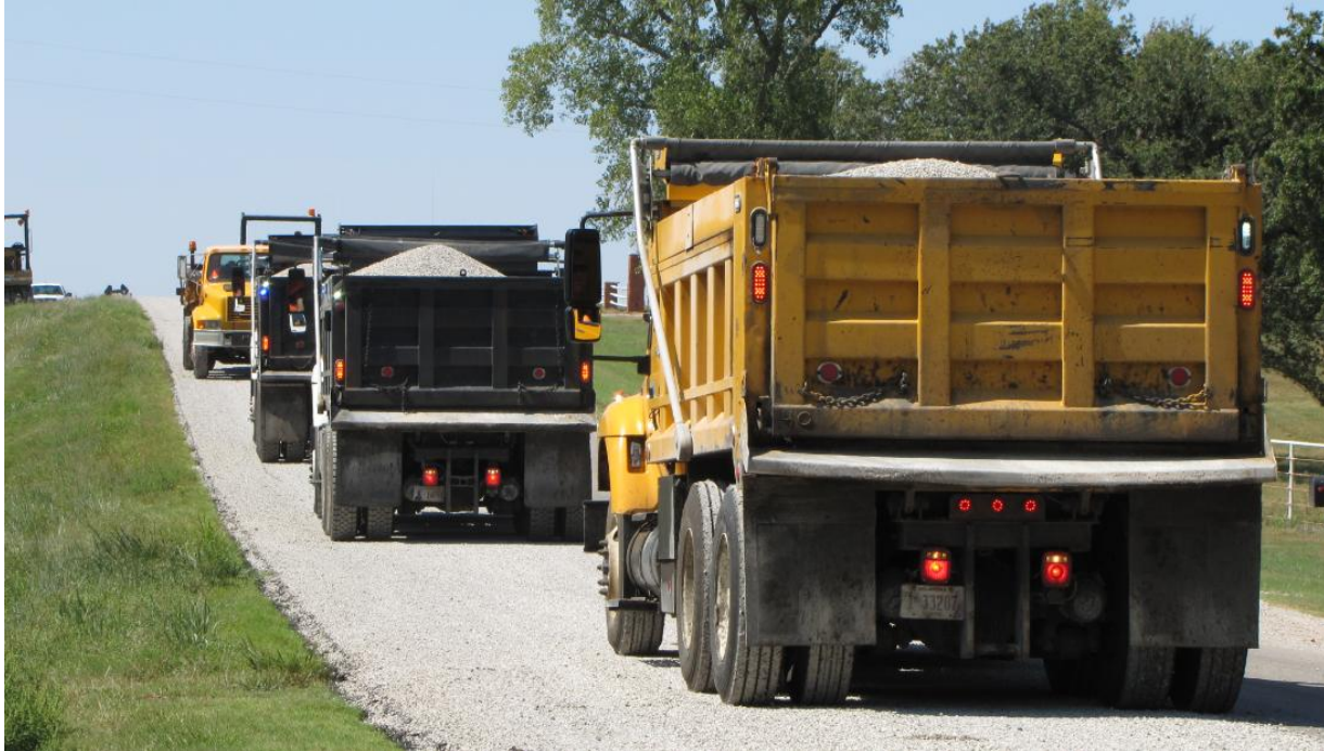
Figure 6.8 Dump Trucks in Staggered Pattern
