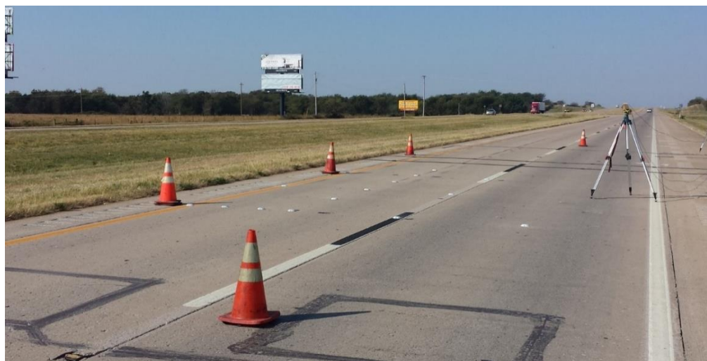
Figure 5-8 Field test 3 deployment site
