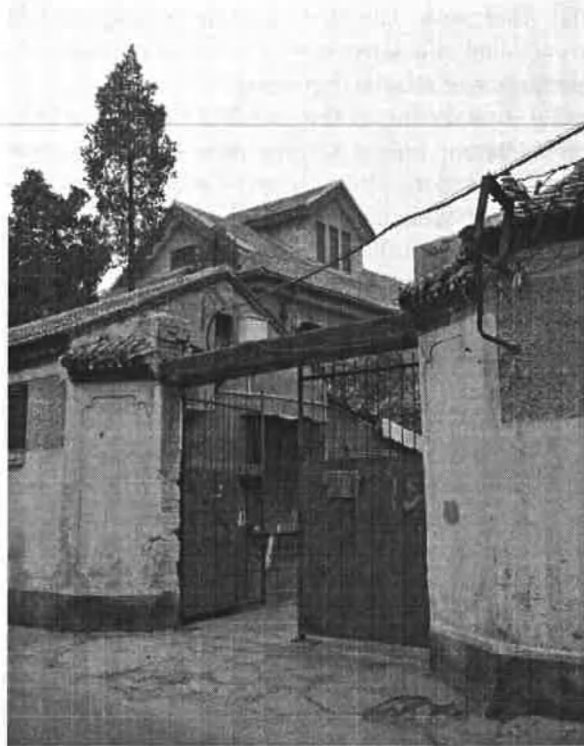
Figure 2: The recent condition of No. 9, Bingmasi (photograph by TANG Wenyu)
