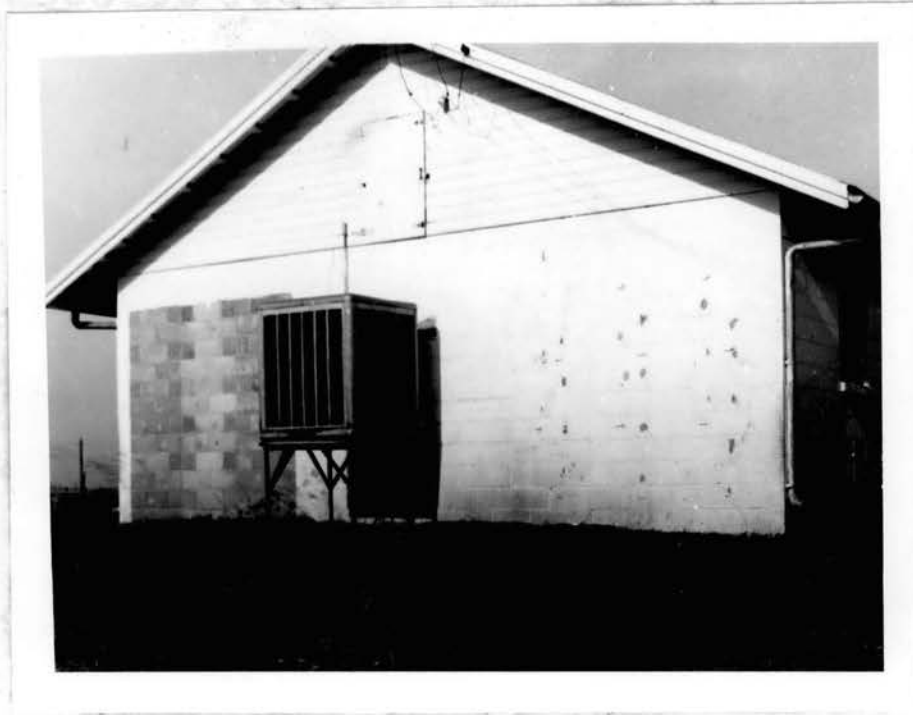
Fig. 2 - West Wall of Temperature-Controlled Shelter Showing the Unpainted Panel on the North and the Painted Panel on the South.
