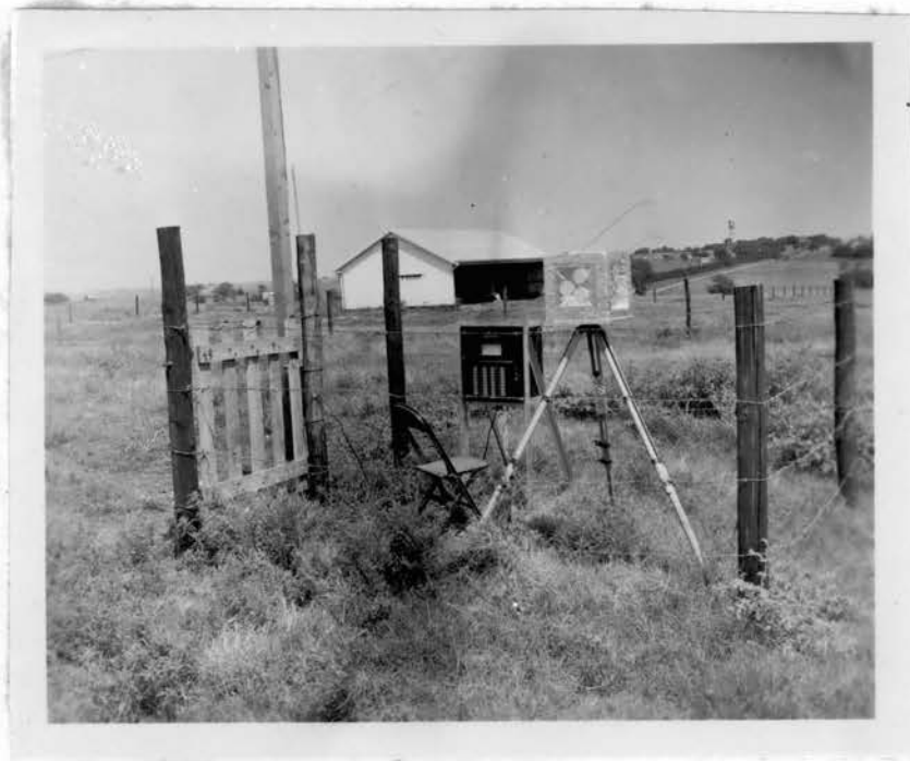
Fig. 18 - Enclosure and Instruments Used in Recording Sol-air Temperatures.
