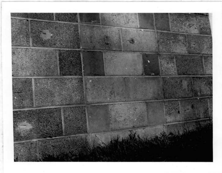
Fig. 14 - Unpainted West Wall Panel in Temperature-Controlled Shelter For Dairy Cattle Showing Shades and Textures of Expanded Shale, Left, Sand and Gravel, Center, and Pumice Aggregate Concrete Block, Right, and Grooves for Thermocouple Junctions.
