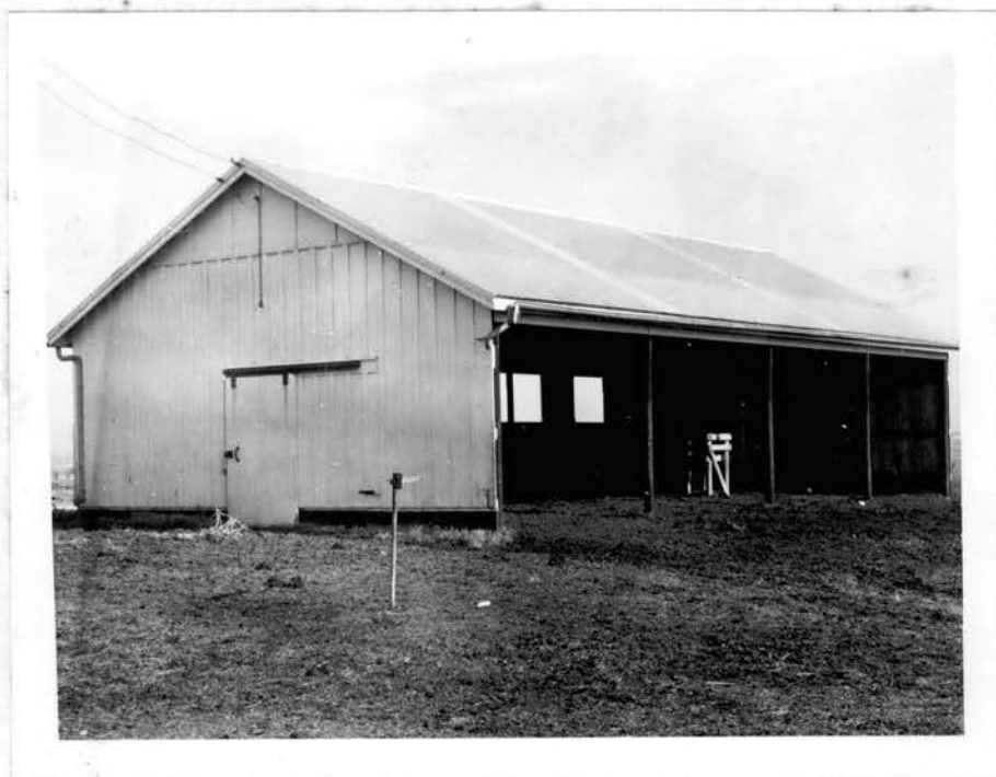
Fig. 13 - Experimental Open Front Shelter for Dairy Cattle Showing Open Front Facing South. Galvanized Roofing Sheets Appear As Two Light Colored Strips on South Slope of Roof.
